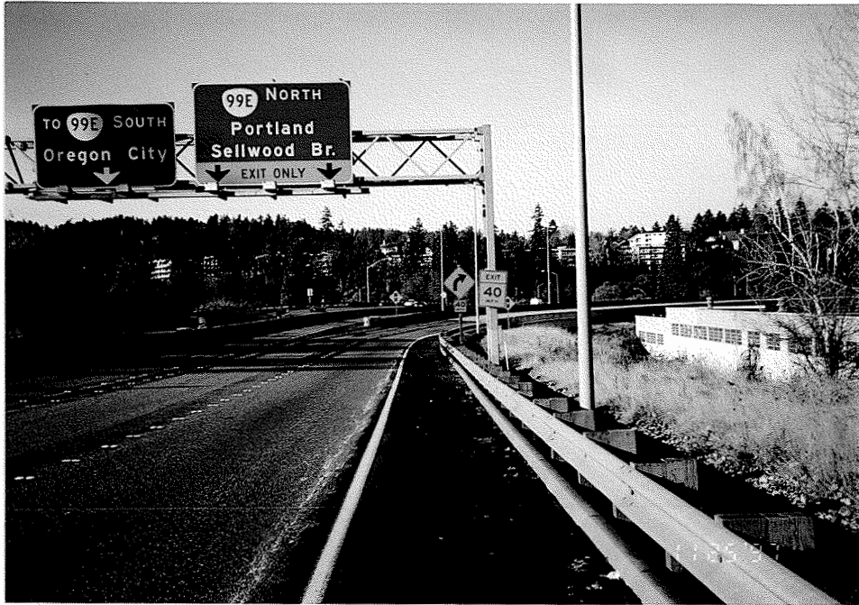
Figure 1.2 Bridge # 9669A, south embankment as seen from Ore 224.
