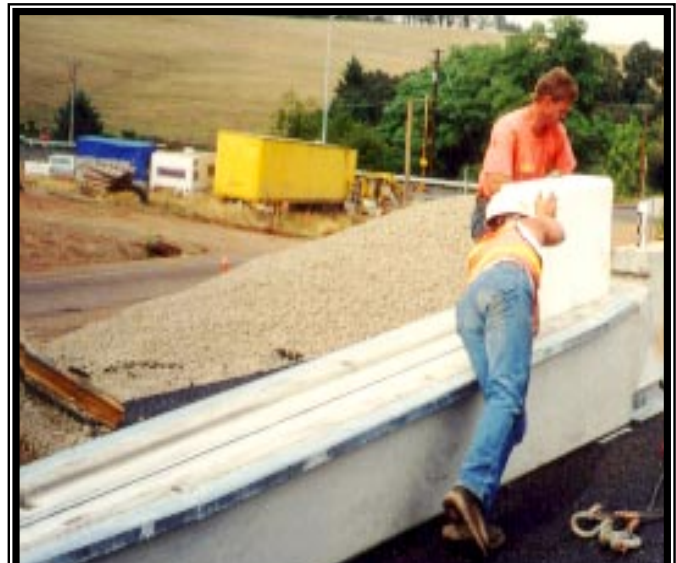
Workers begin fitting the crushable blocks to the base
