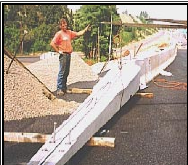
Installation of the wedge shaped end terminal base
