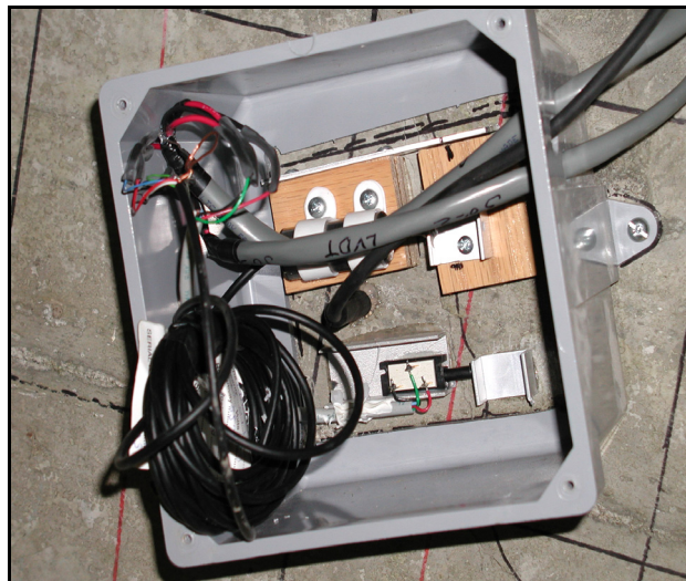
Crack opening and temperature sensors installed on bridges
