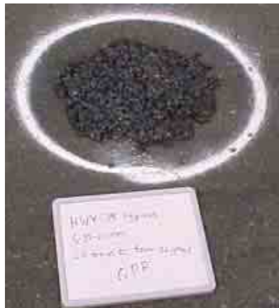
Figure 4.8: QPR2000 metal signal plate patch
