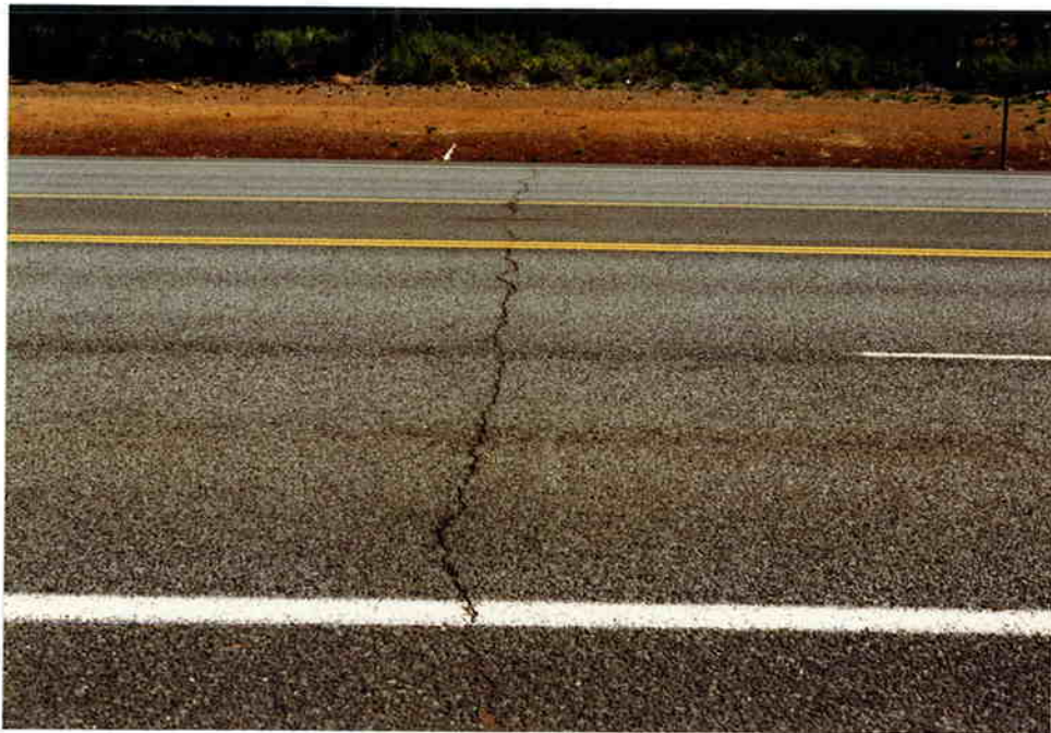
b) Typical Transverse Cracking
