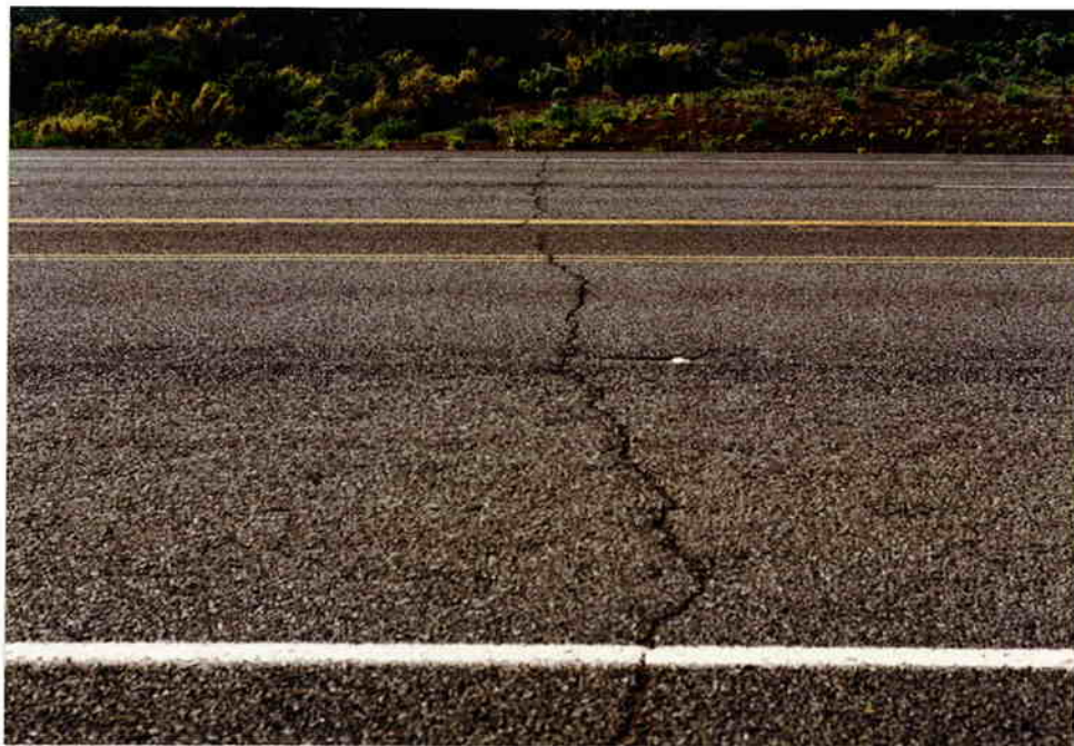
b) Typical Transverse Cracking
