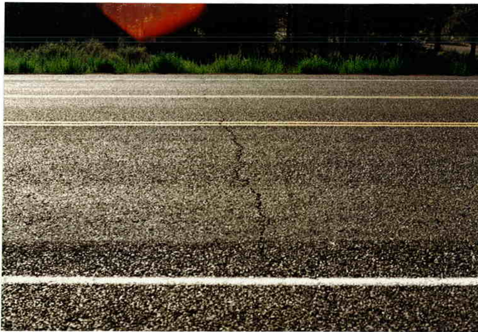
b) Typical Transverse Cracking
