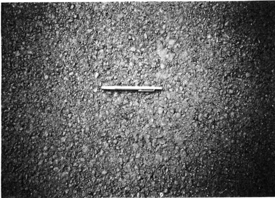
Figure 6.6 - Close-up of Fiber Pave, MP 150.62
