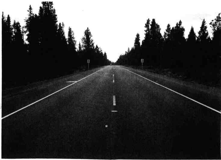
Figure 6.7 - Typical Pavement Condition of Control with Lime (right) and Class "C" with Pave Bond (left), MP 160.21
