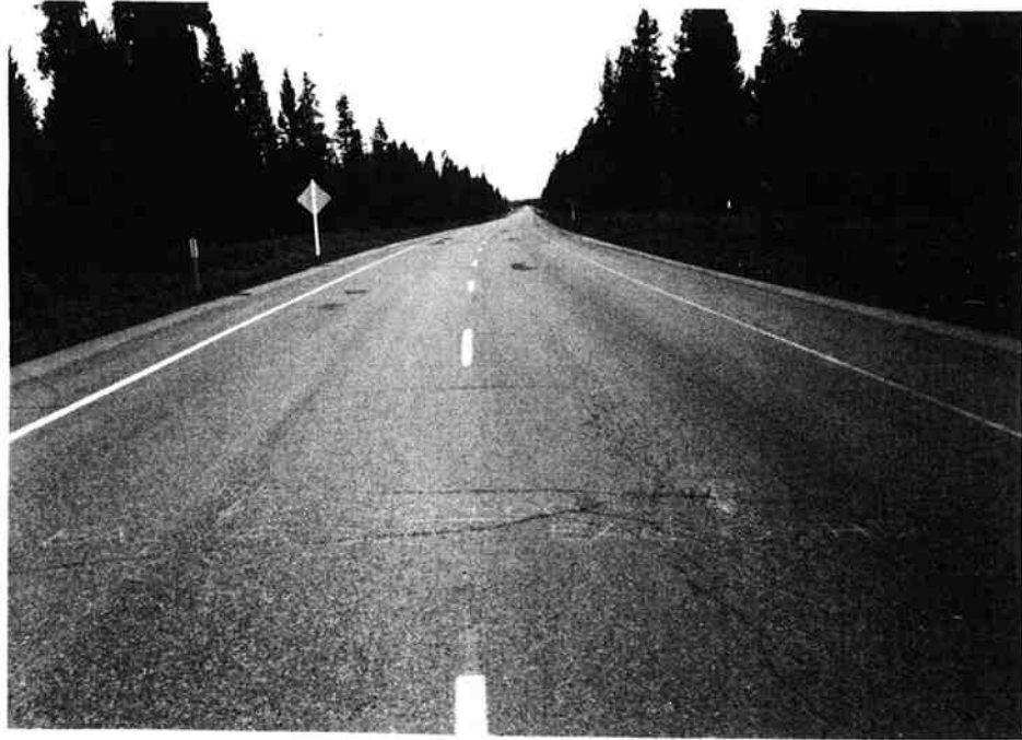
(a) MP 161.02 Facing South
