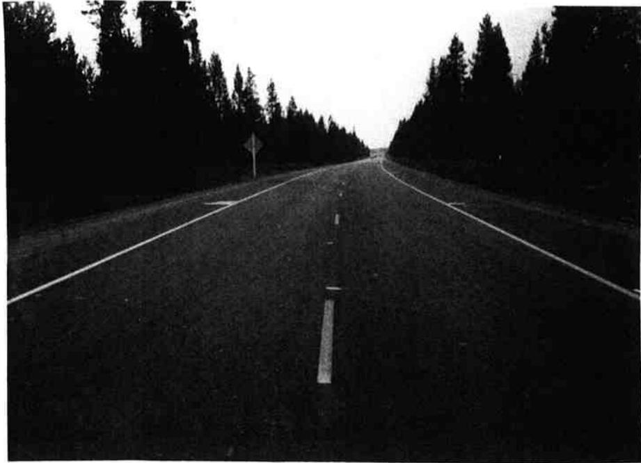
Figure 6.9 - Typical Pavement Condition of Control (right) and Class "C" with Lime and Pave Bond (left), MP 161.02
