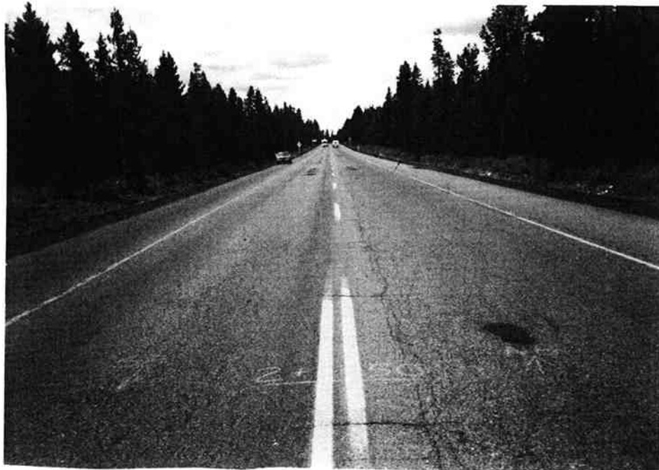
(b) MP 160.26 Facing North
