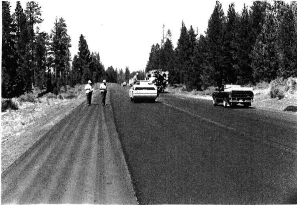
(a) Vibratory Roller
