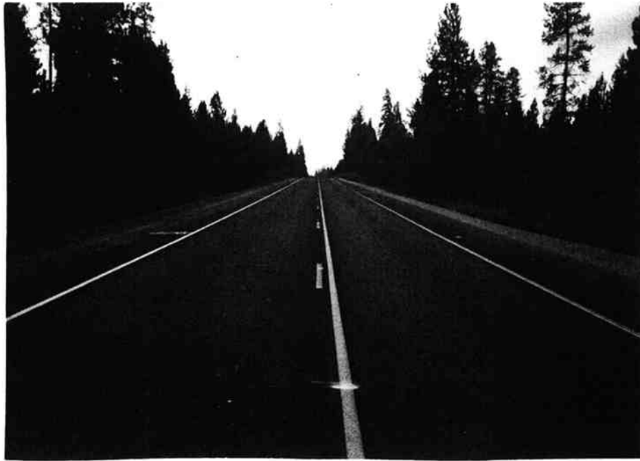
Figure 6.1 - Typical Pavement Condition of PlusRide after Overlay, MP 158.21, Looking South
