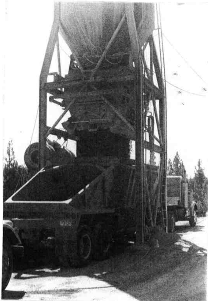
Figure 4.6 - Depositing Mix into Truck
