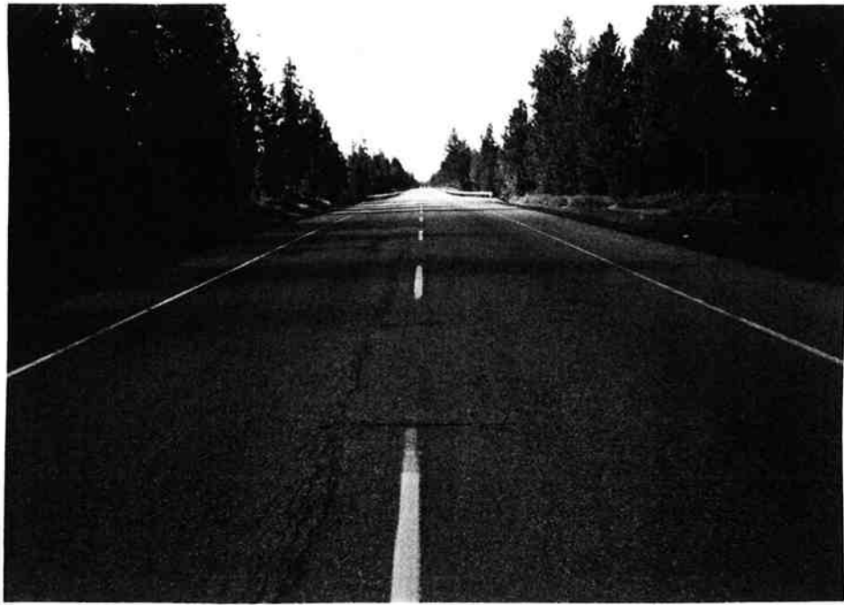
(a) MP 159.62 Facing South
