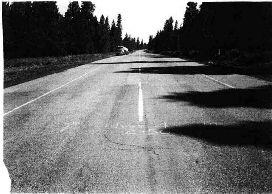
(b) MP 159.67 Facing North
