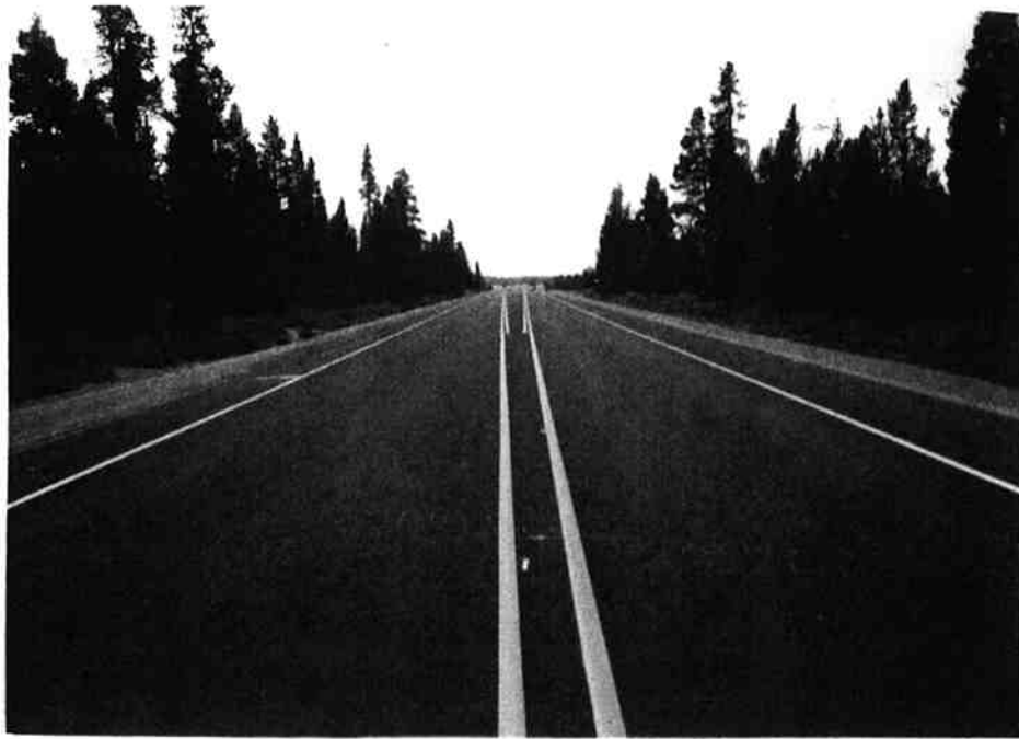
Figure 6.11 - Typical Pavement Condition of CA(P)-1, MP 161.46, Looking South
