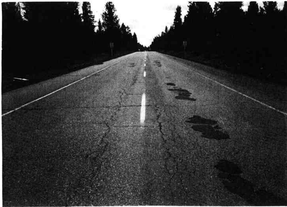
(a) MP 160.21 Facing South
