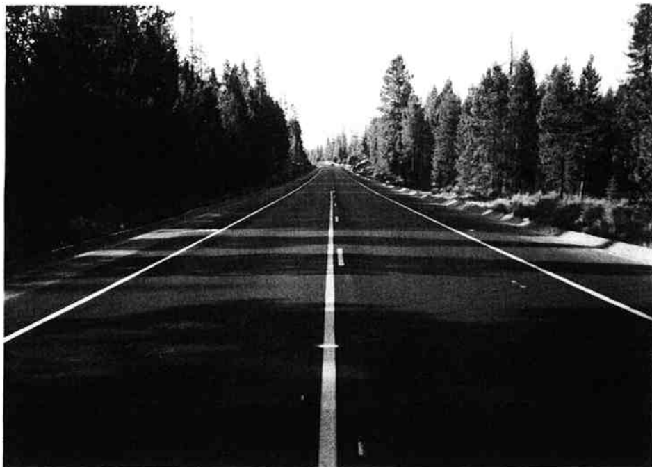
Figure 6.2 - Typical Pavement Condition of Arm-R-Shield after Overlay, MP 158.62, Looking South
