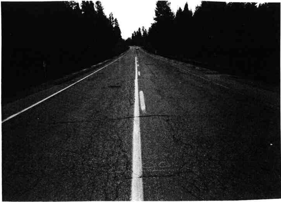
(a) MP 158.62 Facing South
