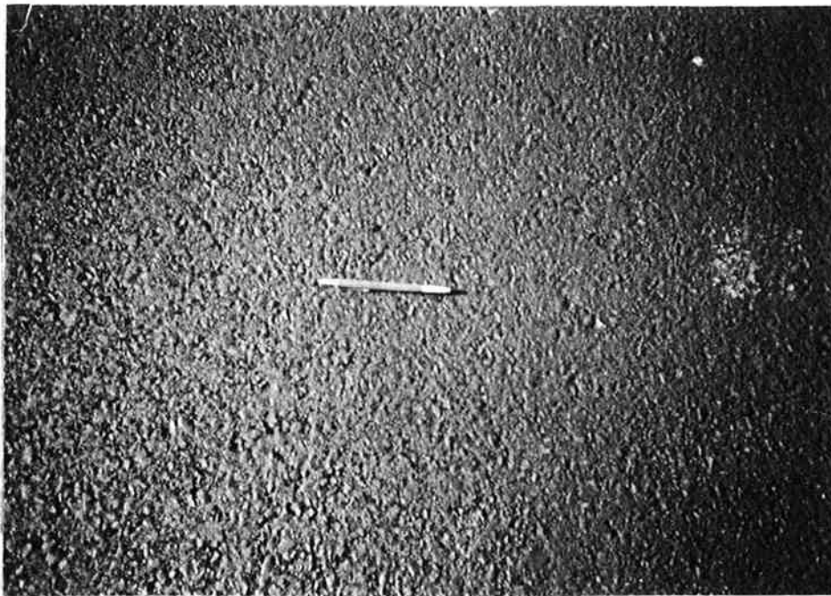
Figure 6.4 - Close-up of Arm-R-Shield, MP 158.62, SB
