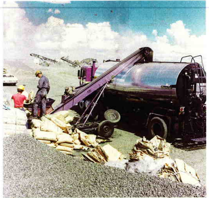
b. Loading Rubber into Distributor
