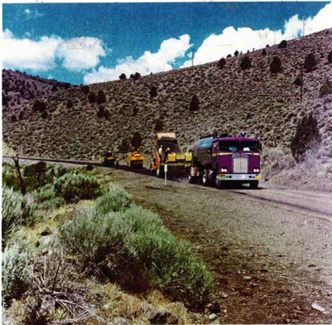
c. Equipment Train: Distributor, Chip Spreader, Rollers
