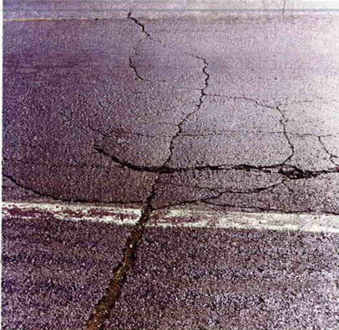
a. Close-Up of Old Pavement
