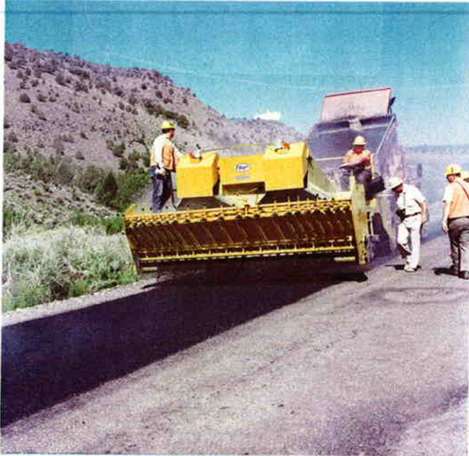
e. Applying Aggregate
