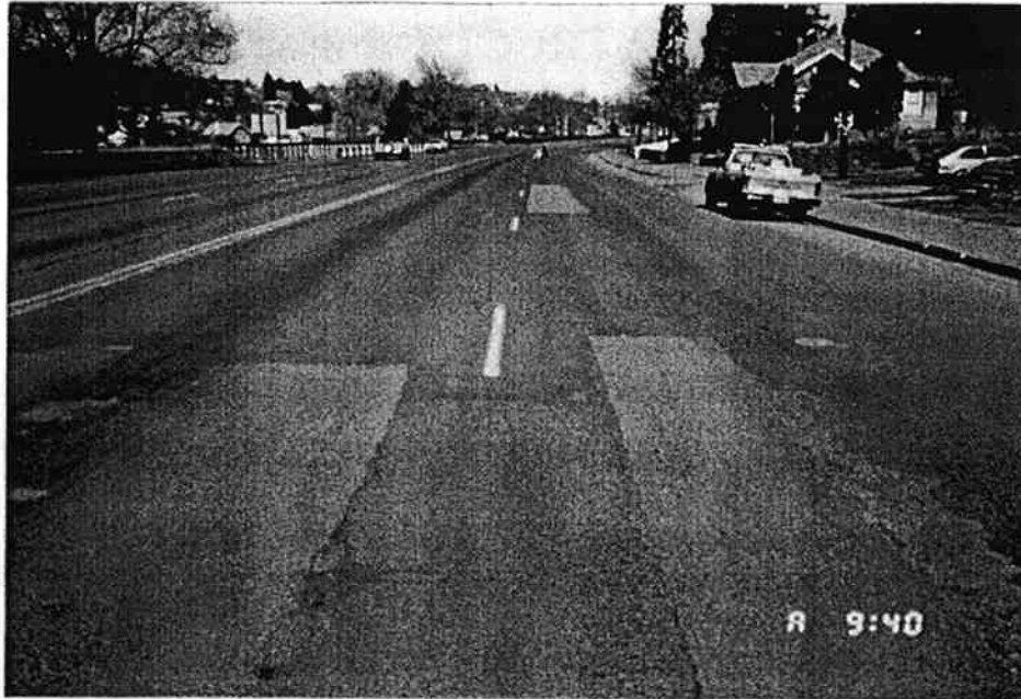
Figure 5.1(b): State Route 39, Northbound at M.P. X5.00 (Prior to construction)
