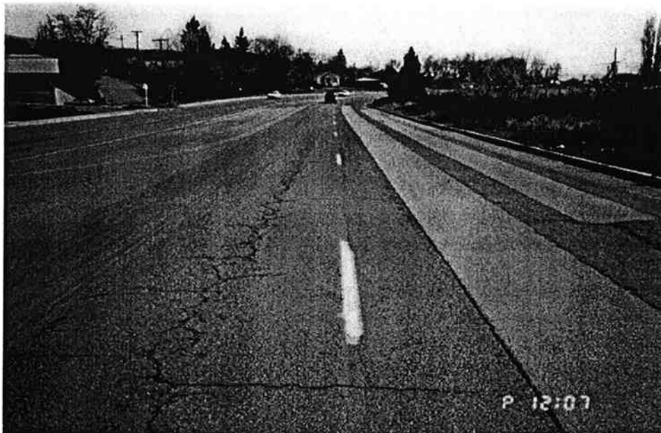
Figure 5.1(c): State Route 39, Southbound at M.P. X4.62 (Prior to construction)
