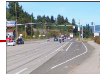
Traffic signal has good visibility for northbound approach.
