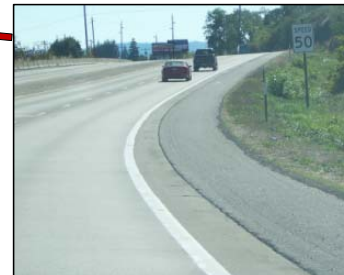
Horizontal and vertical curvature limit sight distance ~1600ft before intersection.
