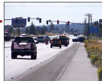
Traffic signal has good visibility from both directions
