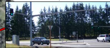
Both minor approaches have sharp curves leading into the intersection (supplemental signals provided)
