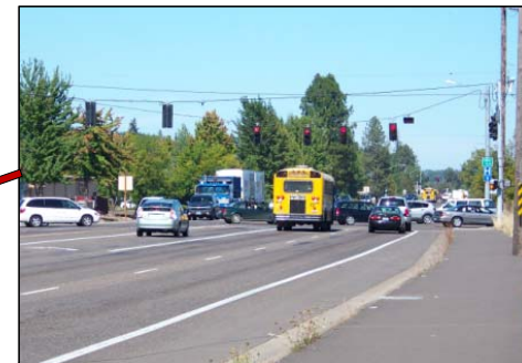
Traffic signal has good visibility
