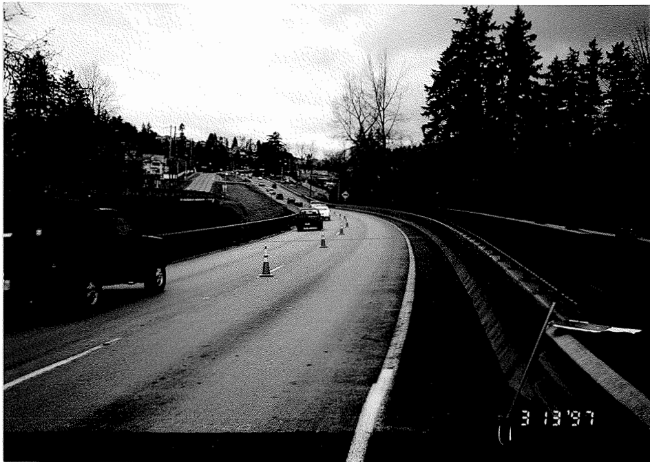
Figure 1.1 The Tualatin River Bridge.
