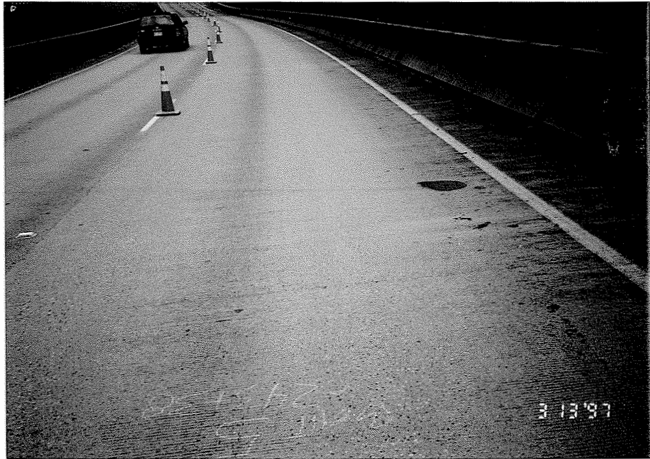
Figure 5.2 Bridge #1417N, most of the deck is in good condition.
