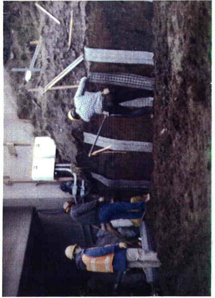
Placing prefabricated drainage liner and chicken wire mesh prior to stabilizing the open face with a temporary flashcoat of shotcrete.
