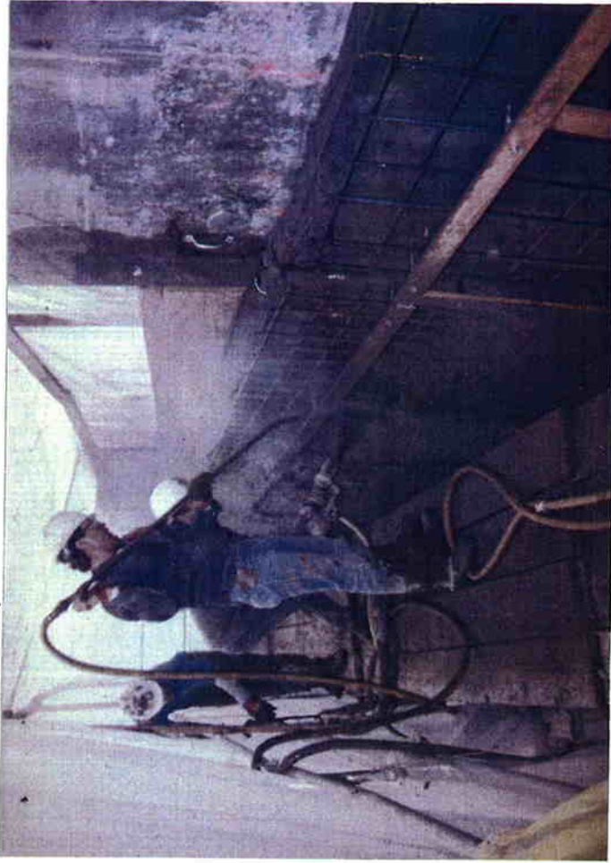
Placing the second shotcrete application (4.5 inches thick) under protective cover.
