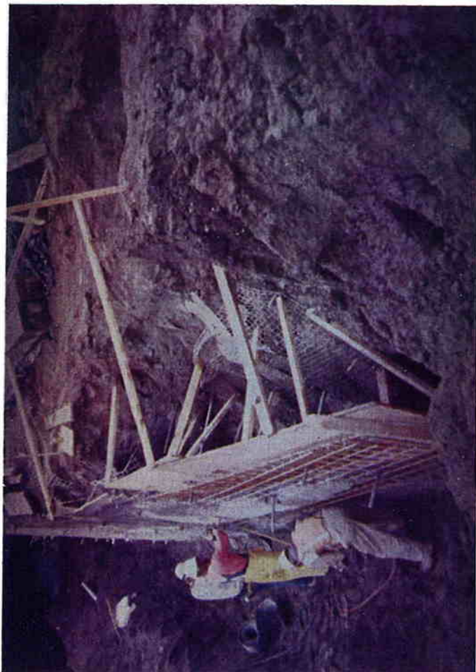
The Contractor formed the wall at the collapsed section, drilled through the forms to install temporary casings, pressure grouted the permanent nails, erected the welded wire mesh and placed the structural shotcrete facing. A lean concrete mix (one bag cement) was placed behind the forms to replace the collapsed soil.
