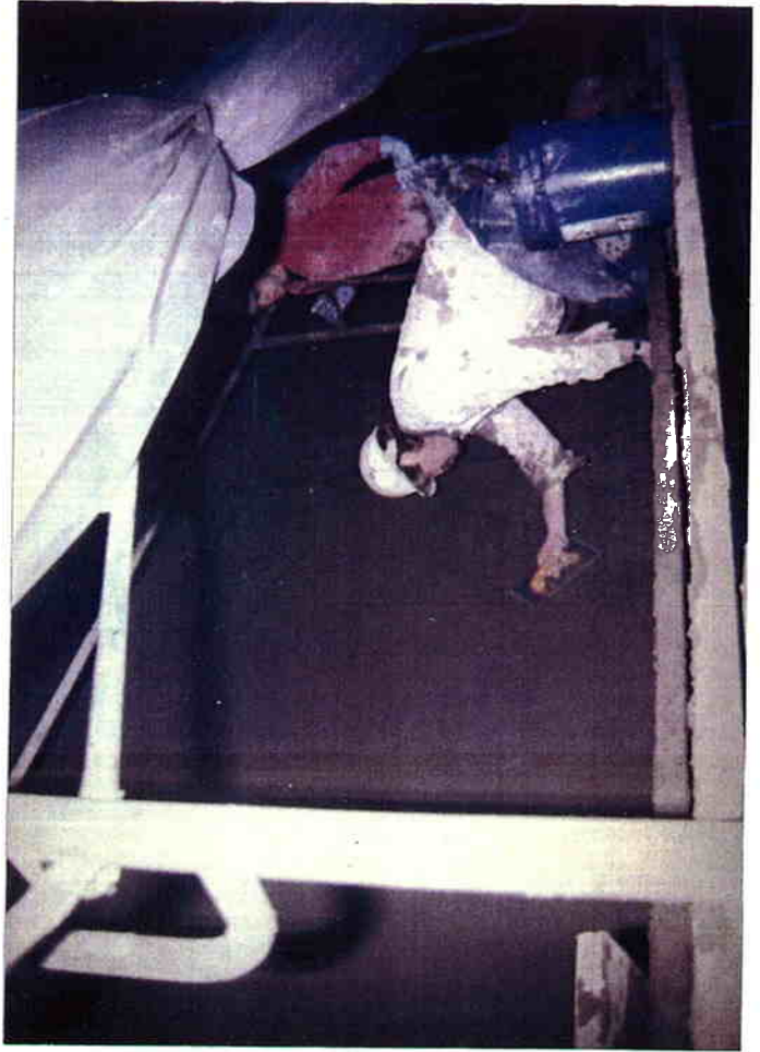
Placing the second shotcrete application (4.5 inches thick) under protective cover.
