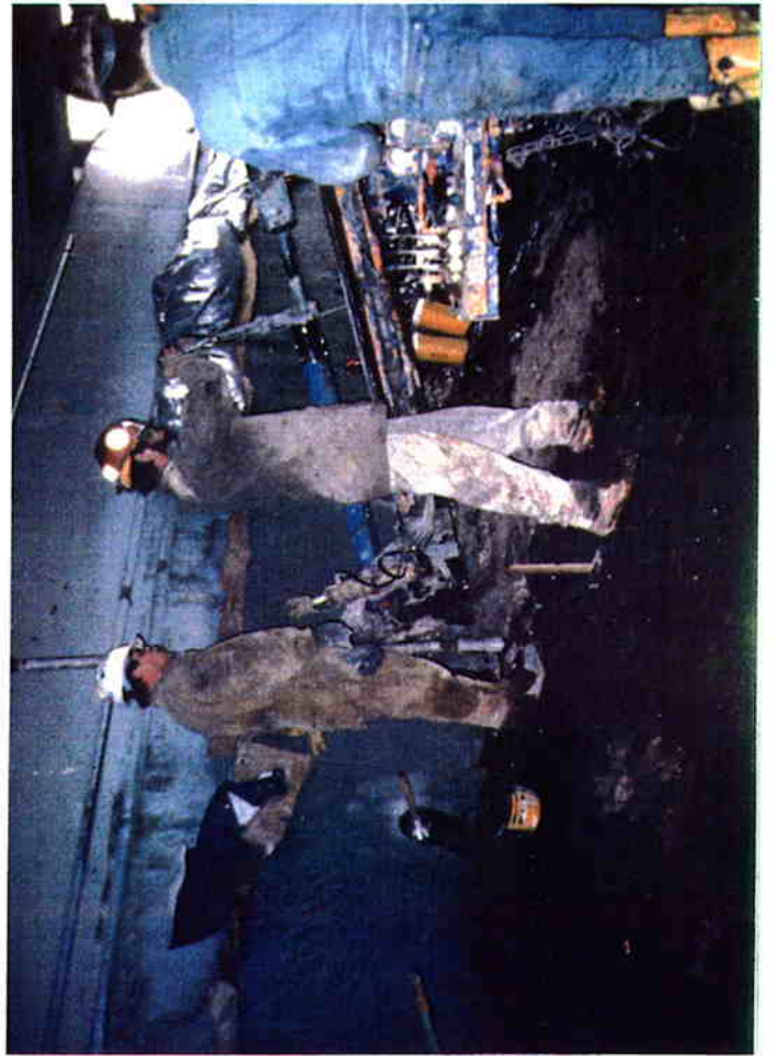
Contractor "braking casing" during the grouting process of the borehole.
