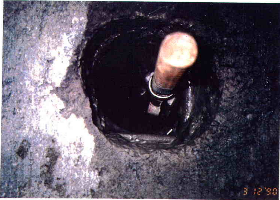
Installed nail following first-stage pressure grouting.
