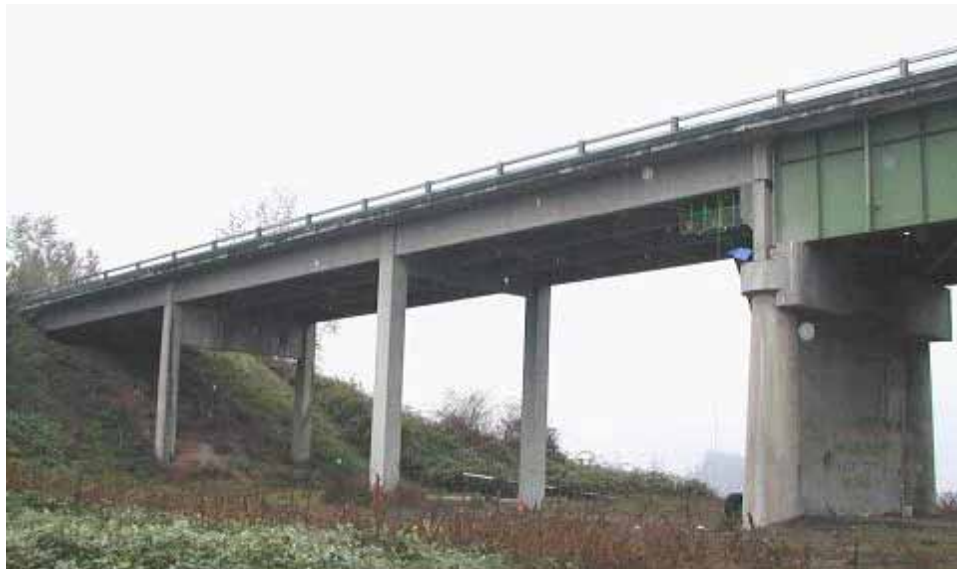
Figure 8.4: South approach spans of Willamette River Bridge on OR 219
