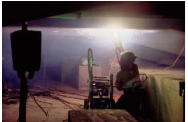
Thermal spraying zinc onto a bridge
