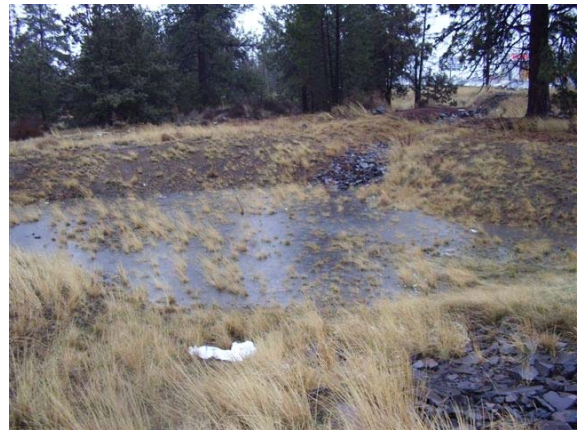
Runoff from U.S. Route 20 during a big rain storm in Bend, Oregon pooling in an ODOT storm water detention pond.
