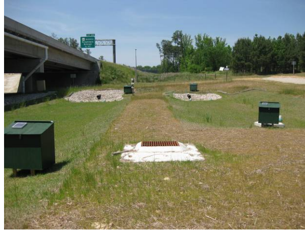
Figure 4. Large (left) and small (right) bioretention basins at Mango Creek.
