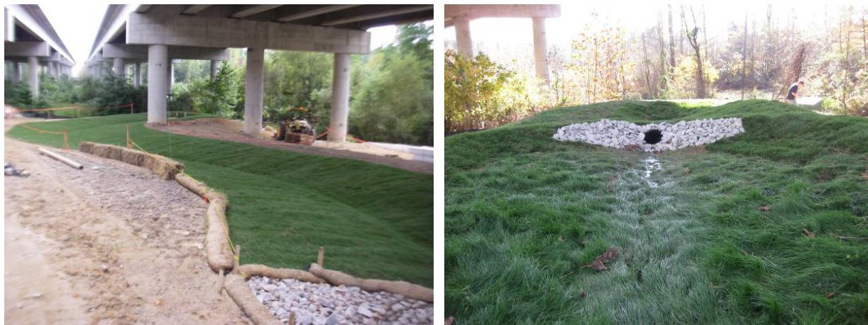
Figure 5. Swale at Mango Creek and the swale outlet pipe.
