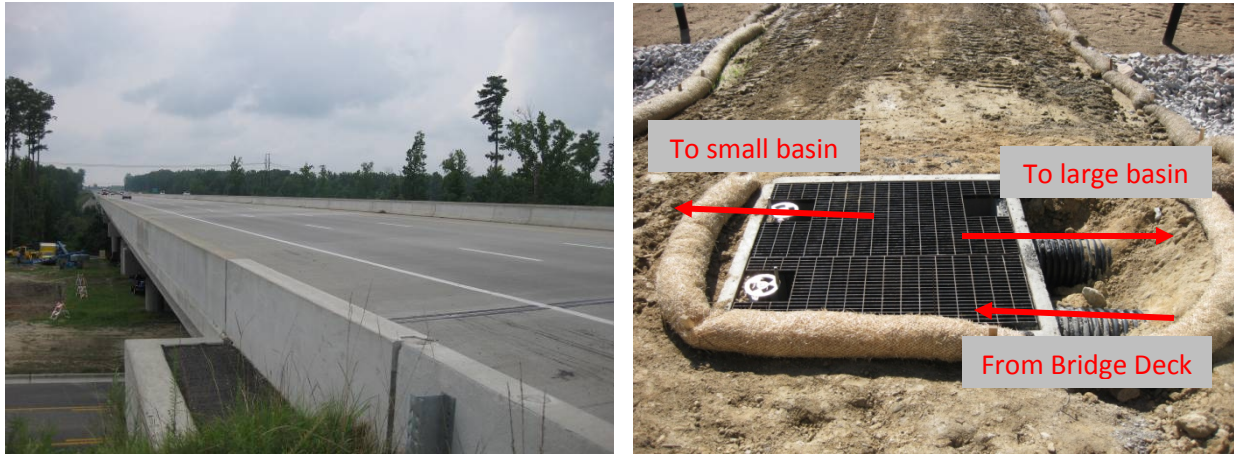
Figure 2. Mango Creek bridge deck (northbound lanes) and distribution box.
