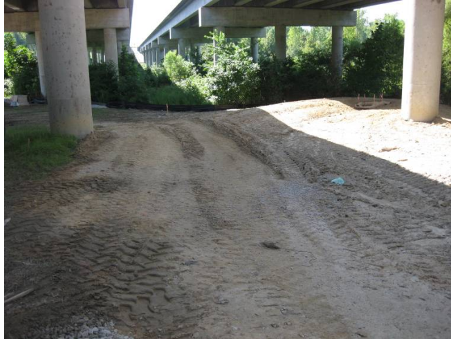
Figure 15. Soil compaction in Mango Creek swale.
