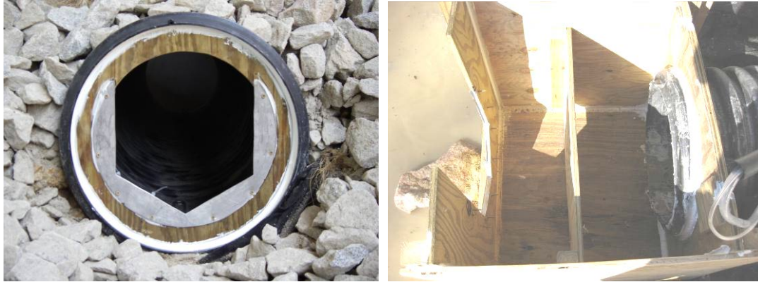
Figure 6. Monitoring installation at inlet (left) and outlet (right) of swale.
