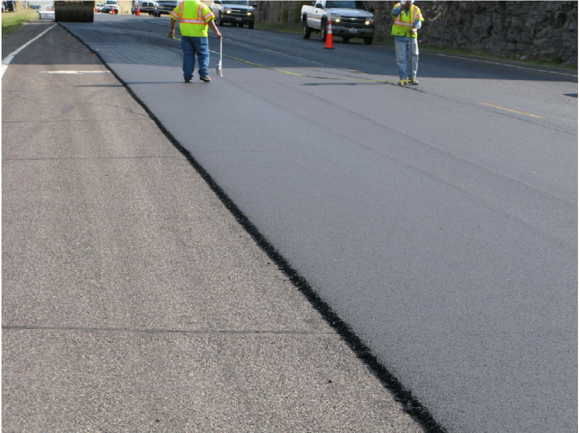
Figure 14. Bumps and Transverse Cracks over Cracks 129, 130, and 131 Northbound US 285
