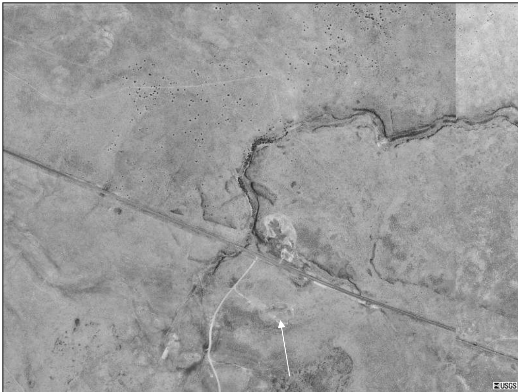
Aerial view of the borrow site in relation to the highway and the surrounding area.
