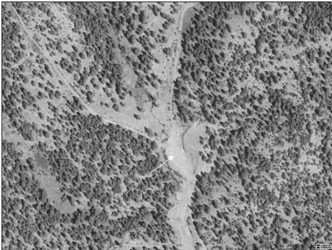
Aerial view of the quarry site along the Forest Service Road.
