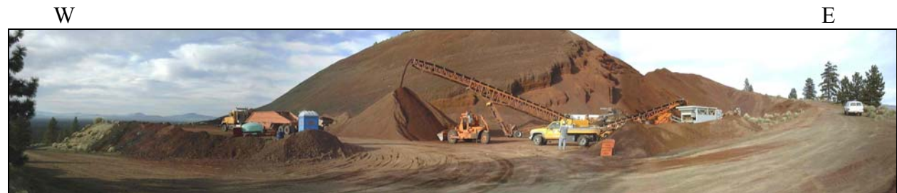
Looking to the north at the process of crushing the cinder at Finley Butte.
