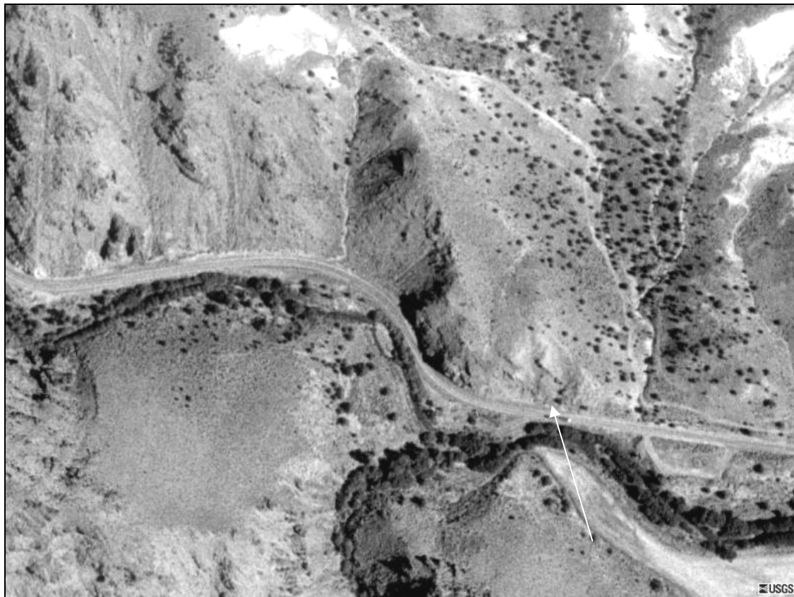
Aerial view of the road cut along the highway.
