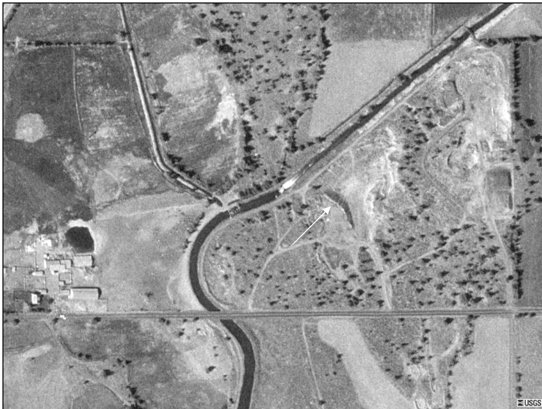
Aerial view of the borrow site located between the irrigation ditch and Young Road.
