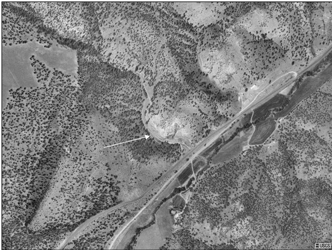
Aerial view of the quarry site along the highway.
