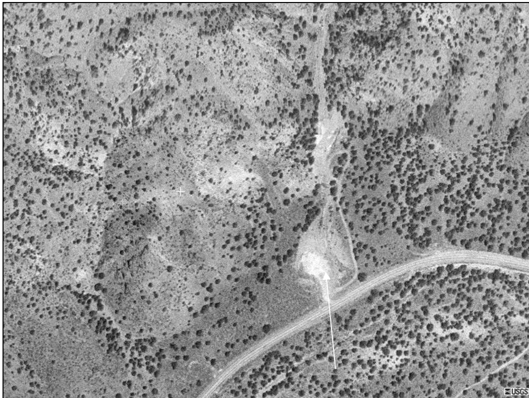
Aerial view of the borrow site at the base of the canyon.
