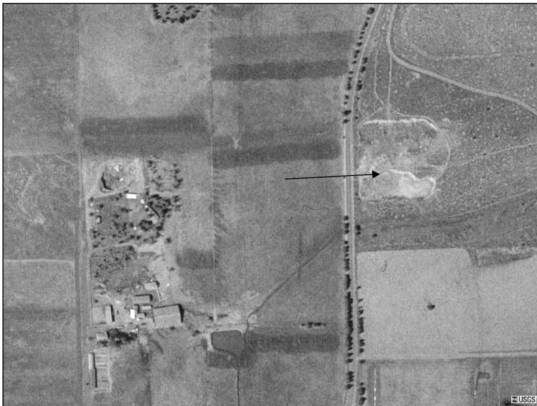
Aerial view of the borrow site in relation to the surrounding property.
