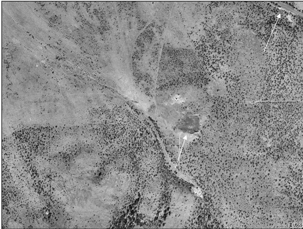
Aerial view of the quarry site, Highway 380 is in the upper right corner.
