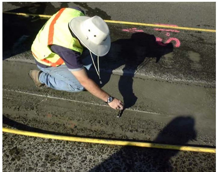
Kevin Haas, ODOT Research Coordinator, verifies the groove depth on one of the concrete test sections
