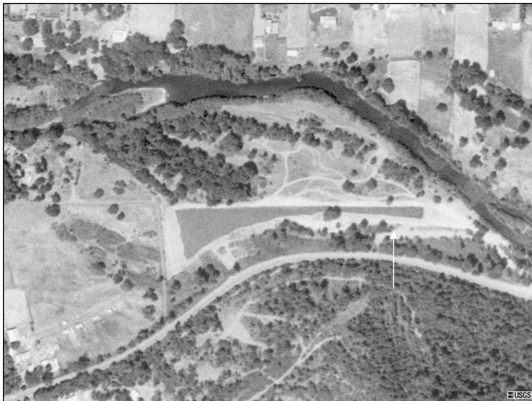
Aerial view of the gravel site along Highway 238.
