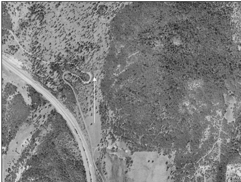
Aerial view of the site in relation to I-5.
