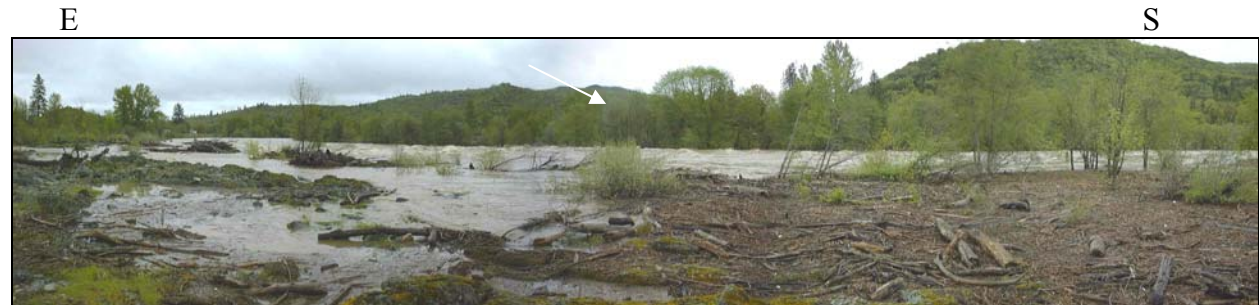
Looking across the Rogue River to the aggregate site.
