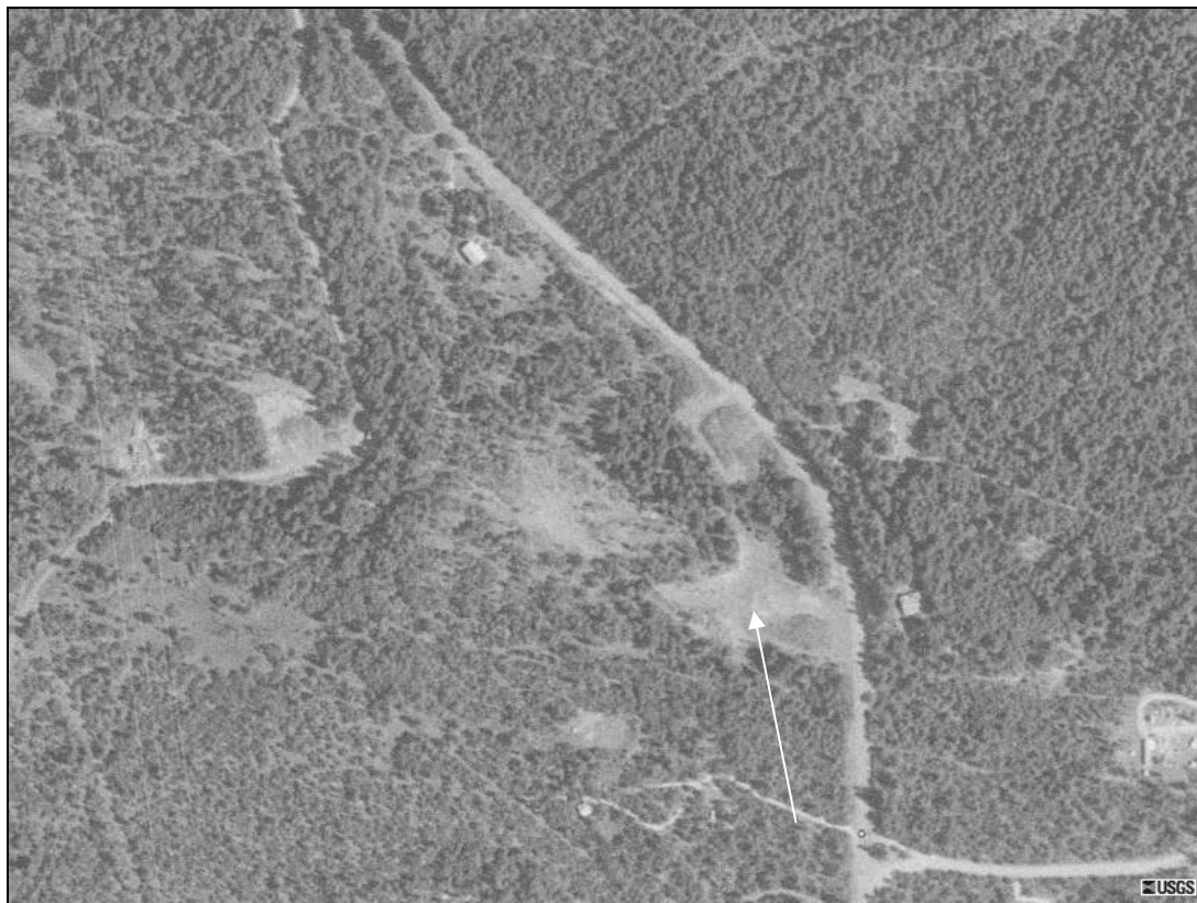
Aerial view of the quarry site along Highway 227
