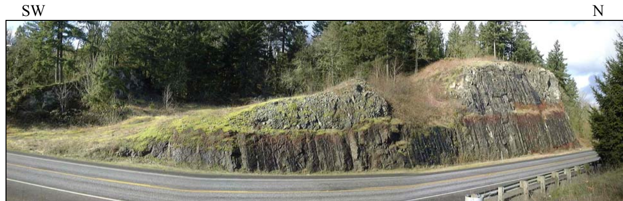
Looking to the west at the property and the road cut along Highway 30.
