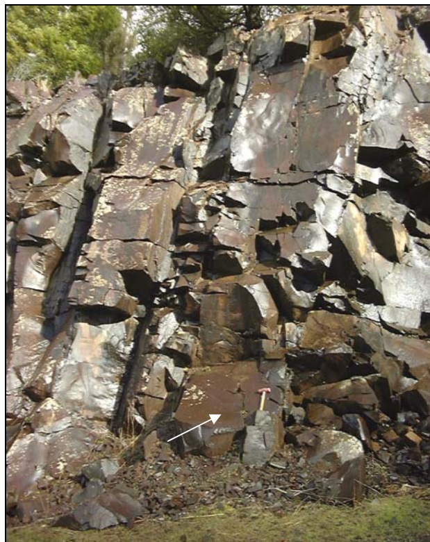
Close-up view of the fracture pattern with the hammer for scale.
