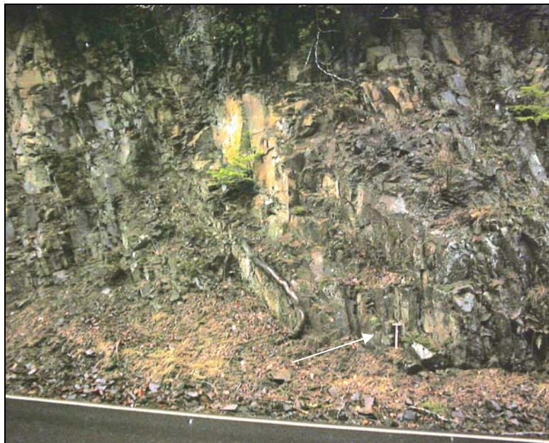
Close-up view along Highway 53 of the jointing pattern.
