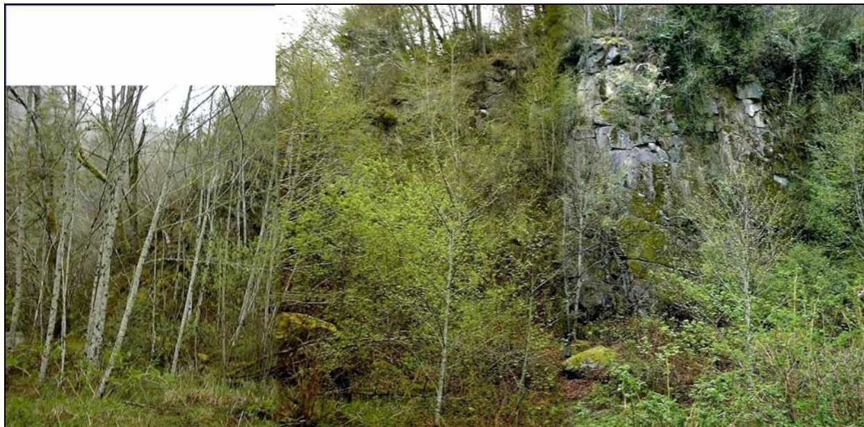
View to the north of the old pit face along the old alignment.
