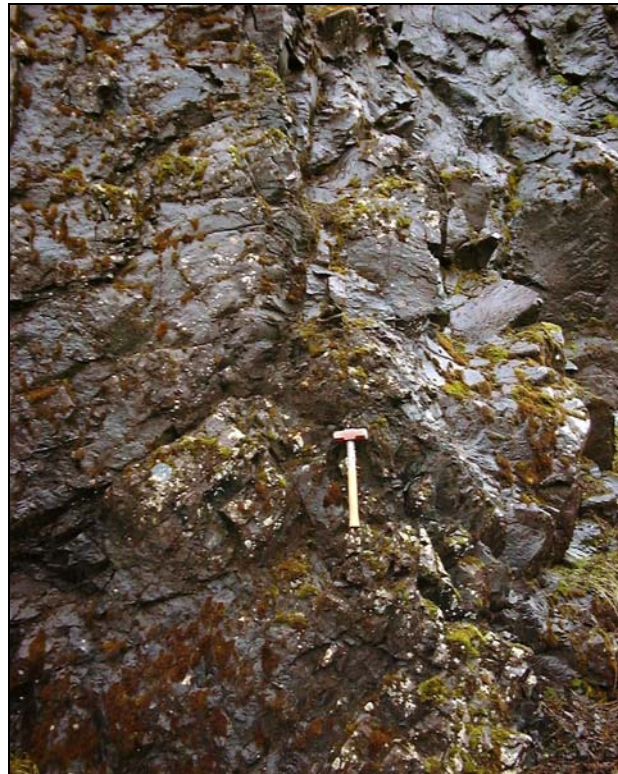
Close-up view of the fracture pattern along the highway.
