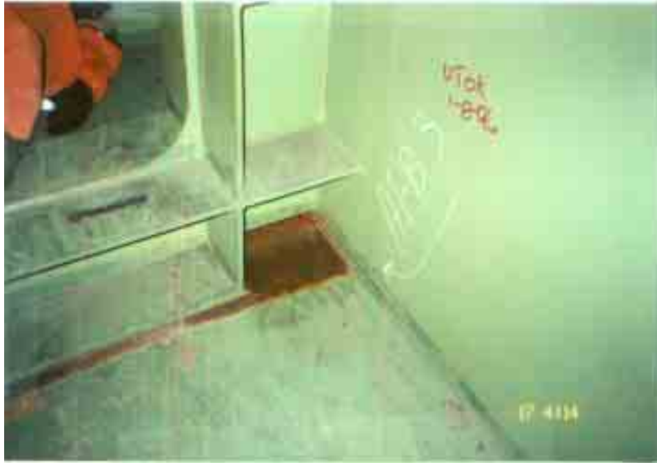
Figure 5.4: Fatigue Category E' detail found in box girders at diaphragm connection to flange. The detail does not effect the butt welds.
