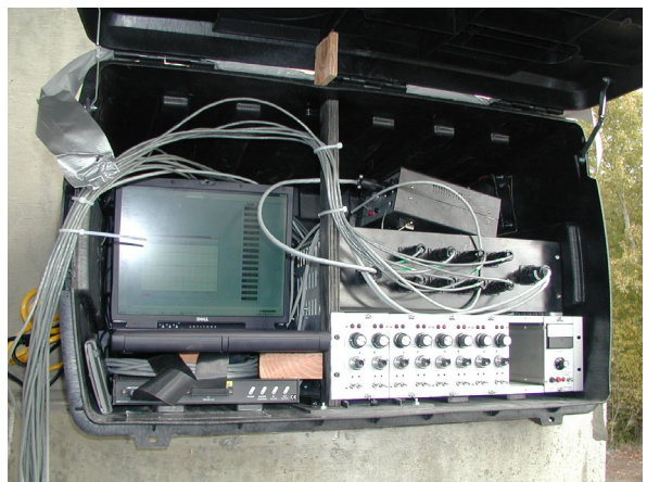
Measurement equipment at Willamette River Bridge
