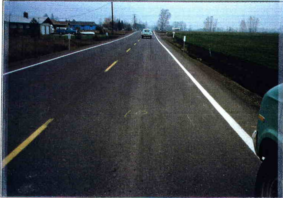
a) At MP 35.00 EB
