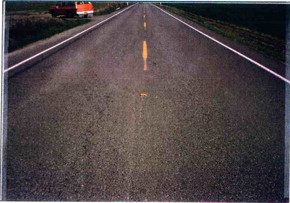
a) At MP 29.63 EB
