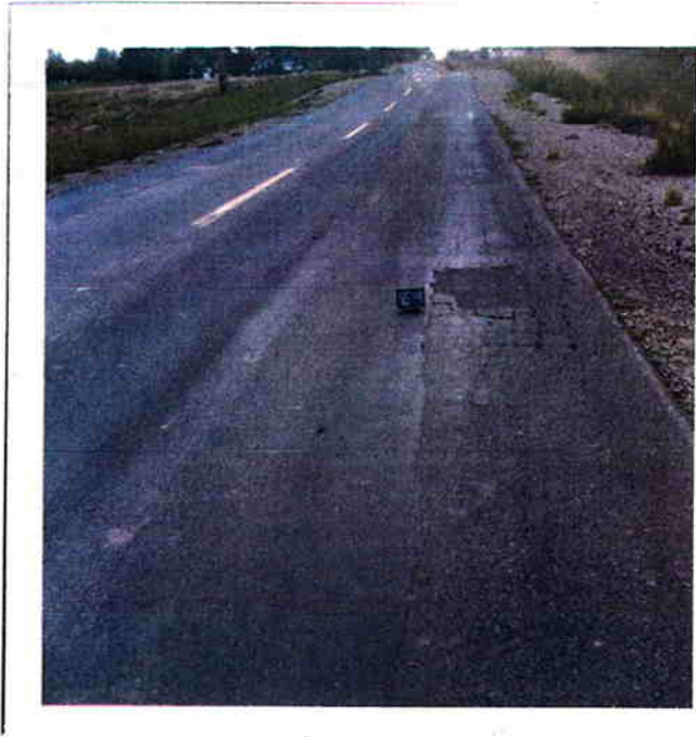
a) At MP 27.00 EB
