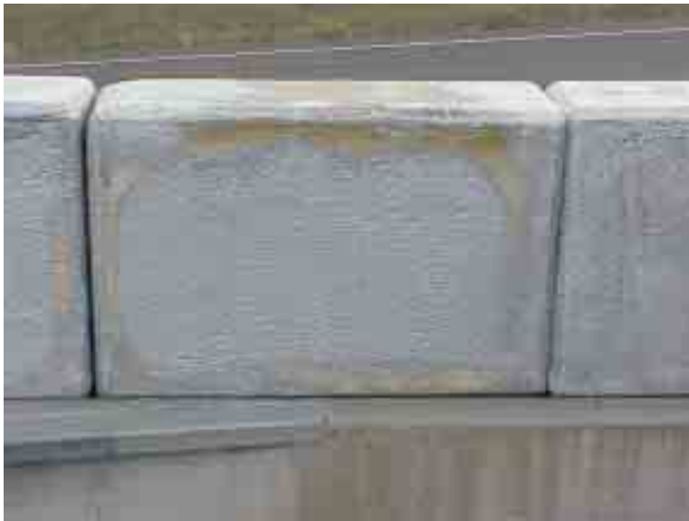
Figure 3.10: Typical Block on Northbound Installation
