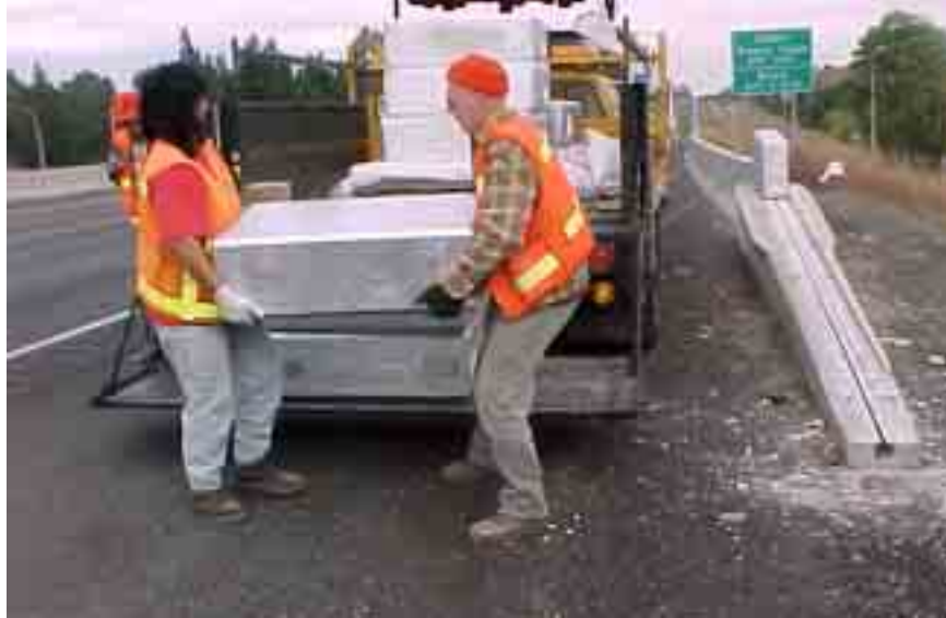
Figure 3.4: Workers Install New Blocks
