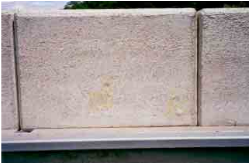
Figure 3.1: Soft Spots on Crushable Block
