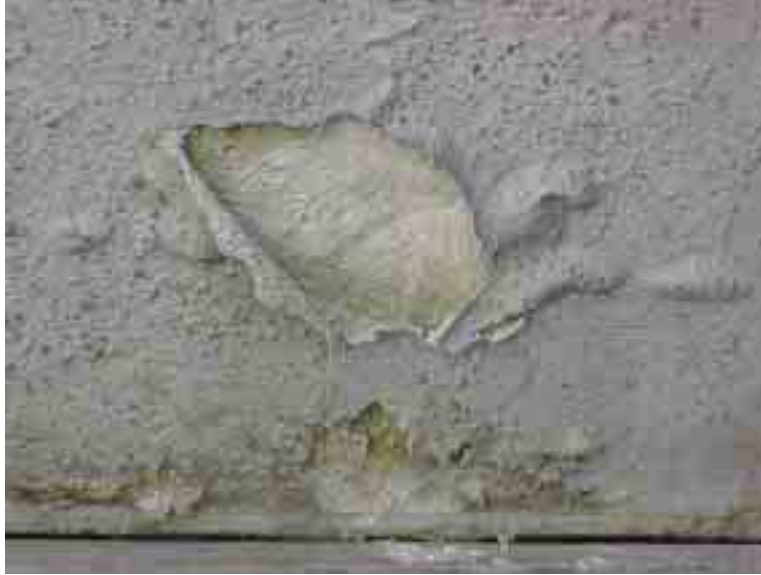
Figure 3.9: Example of Weatherproofing Condition on Southbound Blocks
