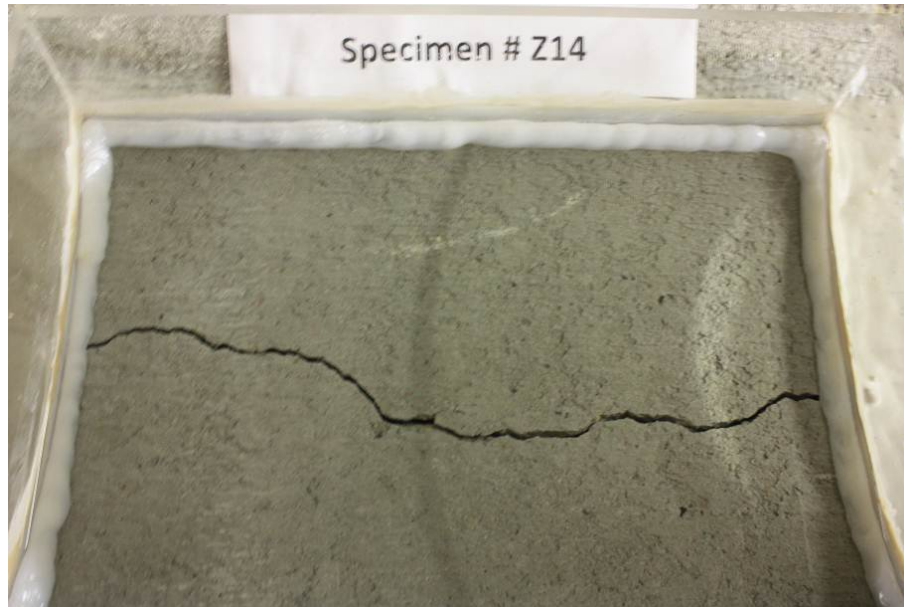
Figure (4.12) Specimen Z14 (0.100-in-wide crack class) showing no corrosion product spots about 52 days after the ponding solution started to incorporate chloride ion
