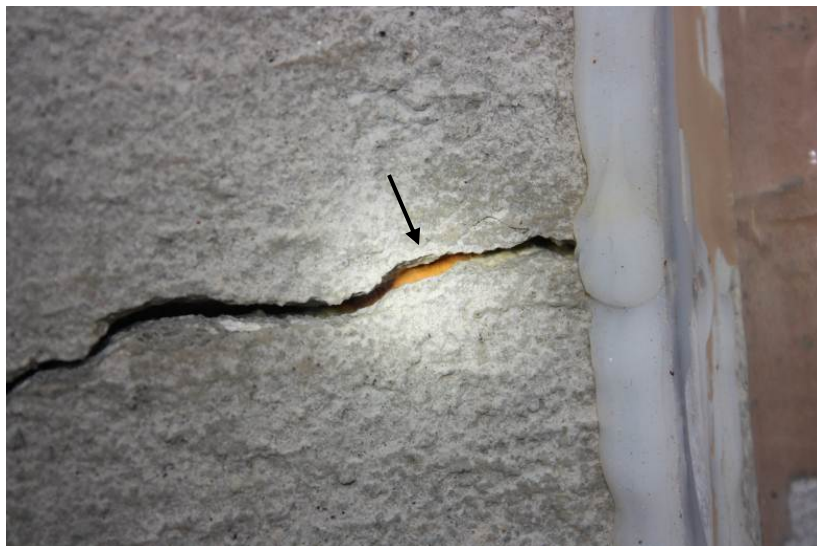
Figure (4.11) Specimen R4 (0.100-in-wide crack class) showing a corrosion spot at a crack-steel wire intersection close to the specimen edge about 52 days after the ponding solution started to incorporate chloride ion
