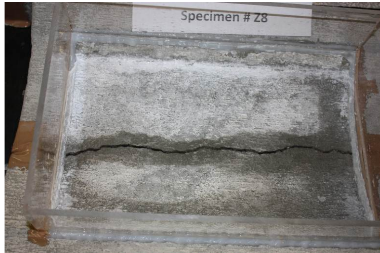
Figure (4.1) Z-type specimen with 0.100-in-wide crack after exposure to saturated calcium hydroxide solution
