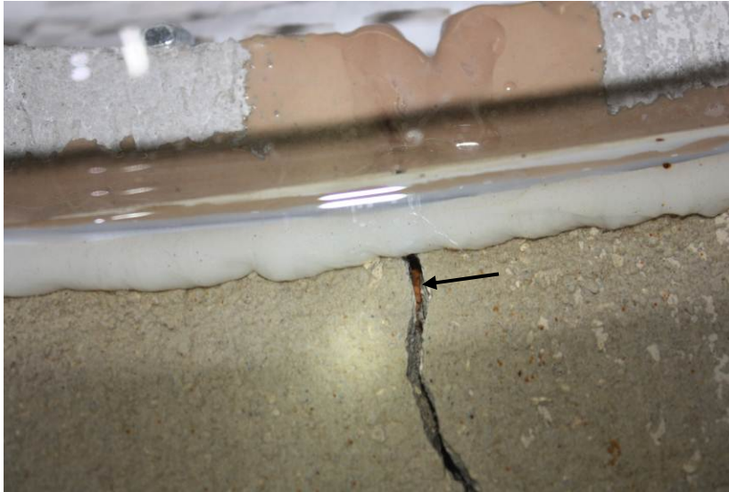
Figure (4.10) Specimen R12 (0.100-in-wide crack class) showing a corrosion spot at a crack-steel wire intersection close to the specimen edge about 52 days after the ponding solution started to incorporate chloride ion
