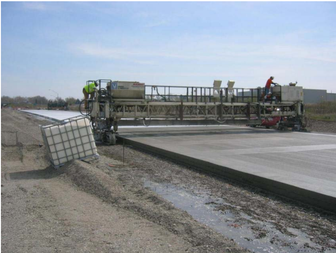
Figure 12. PCC surface tining machine.
