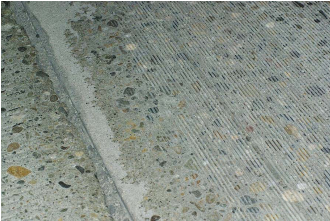
Figure 8. Pavement surface after diamond grinding (right side).
