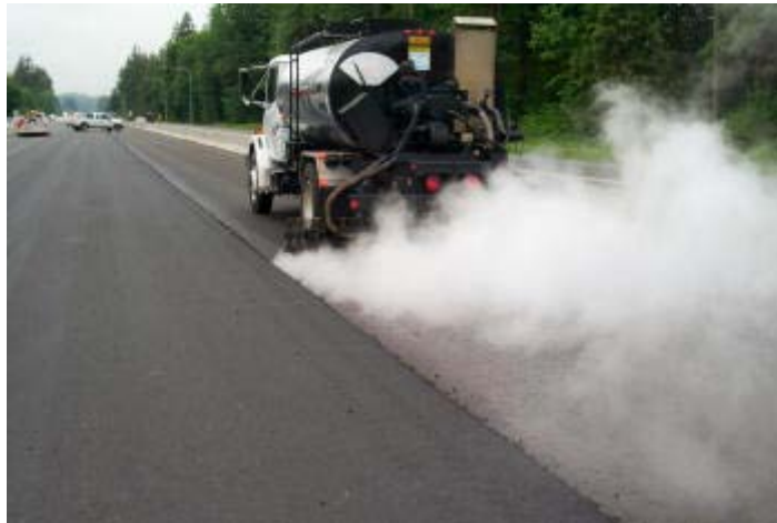
Figure 15. Tack coat application (WSDOT photo).
