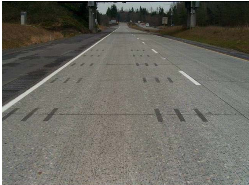
Figure 9. Completed DBR (WSDOT photo).
