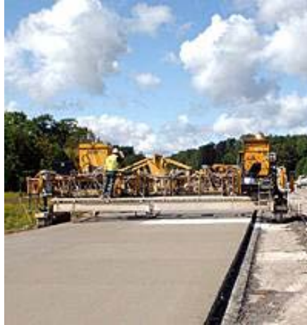
Figure 16: Thin unbonded PCC overlay (Kuennen, 2006)
