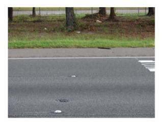
Figure 16 Typical surface holes
