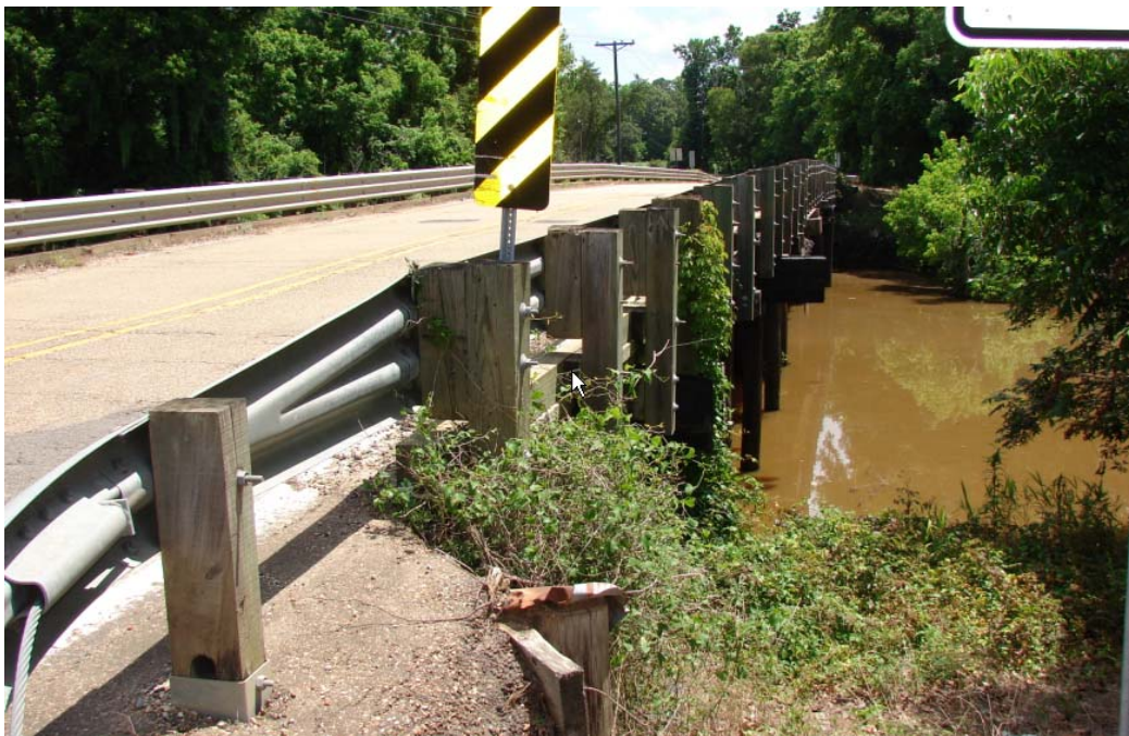
Figure 14 Old Bayou Courtableau Bridge - LA 103
