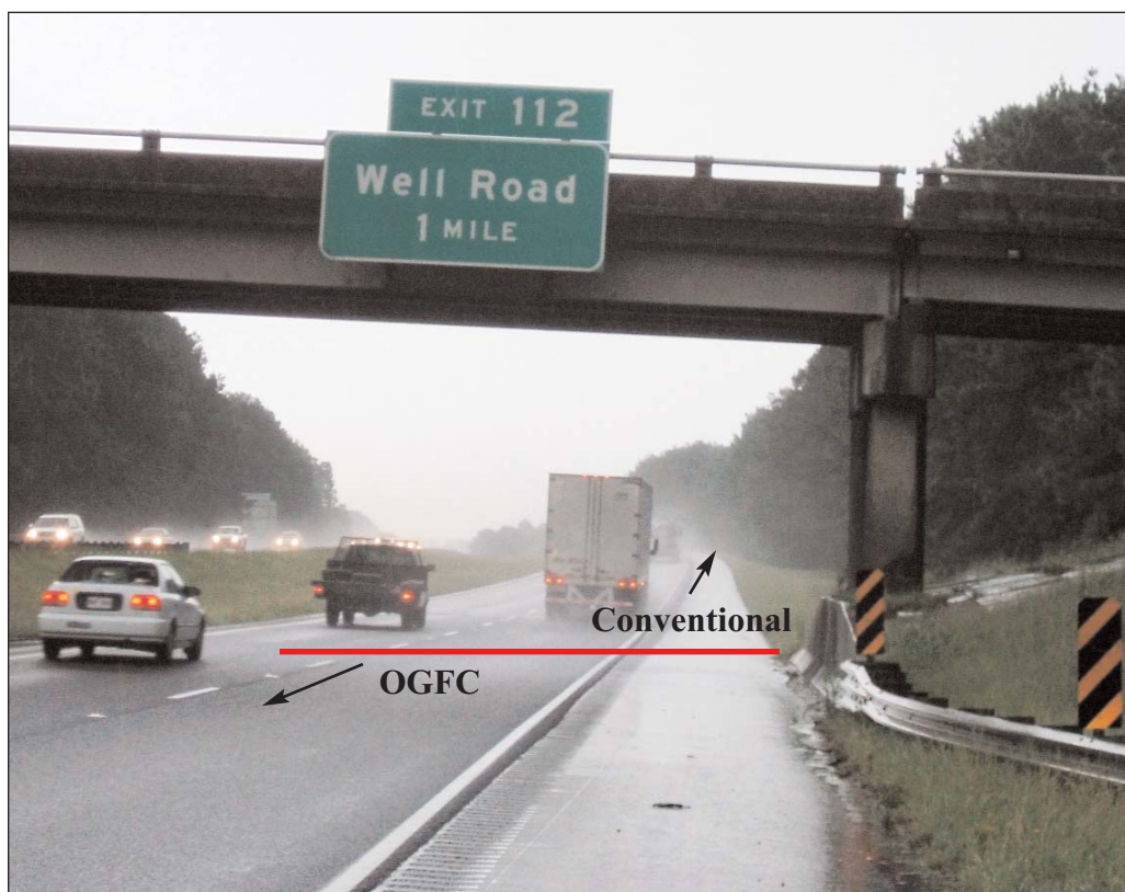
OGFC provides glare and overspray reduction
