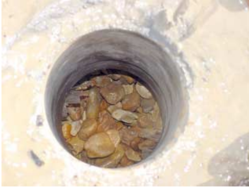
Figure 40 Concrete core hole (US 167 NB, Core N1)
