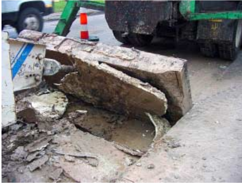
Figure 26 Polyurethane in trenched area (Area 3 Slab 74)
