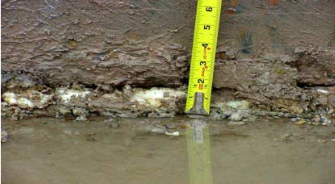
Figure 28 Polyurethane between slab and base course
