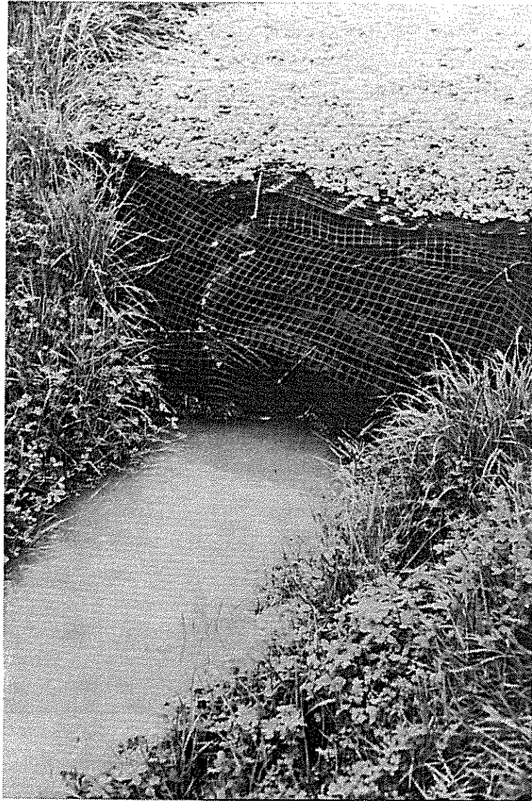
Figure 8. Field installation during a moderate rainfall.
