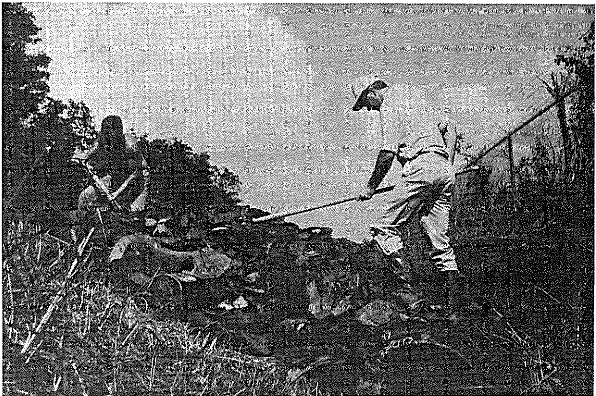
Figure 6. Shredded tires being placed over whole tires.
