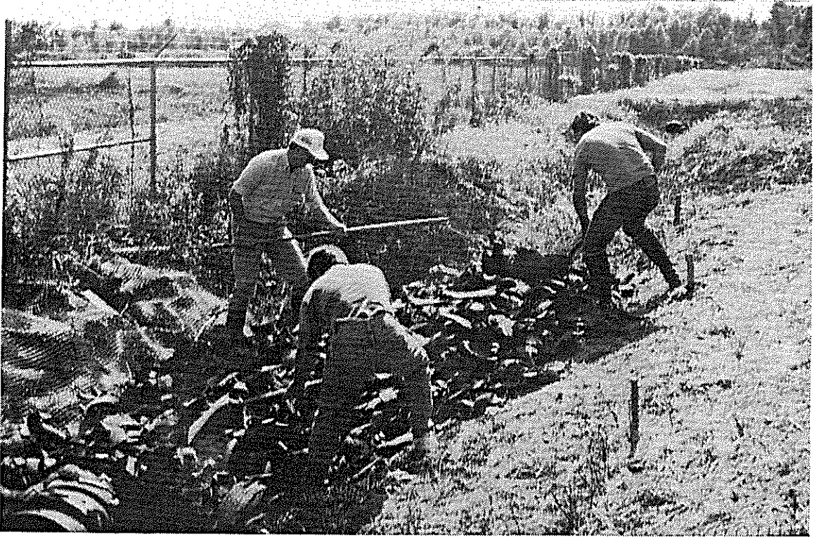
Figure 5. Shredded tires being placed over whole tires.
