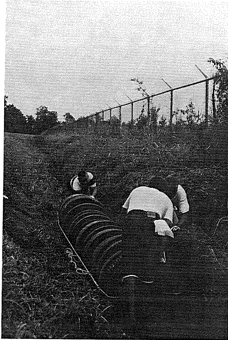
Figure 4. Whole tires installation.
