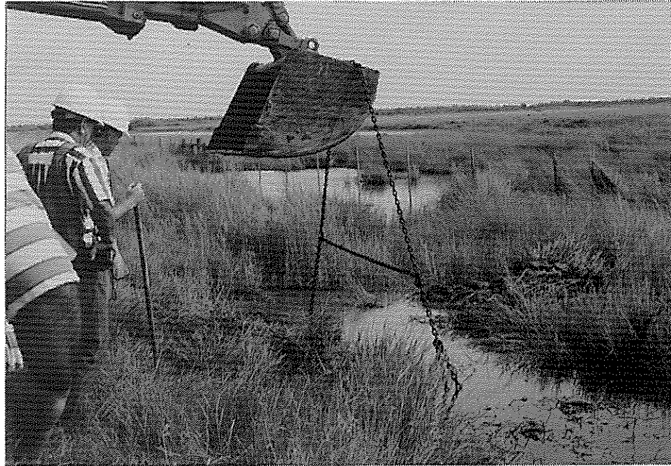
Figure 2. The excavator is seen lifting a culvert.
