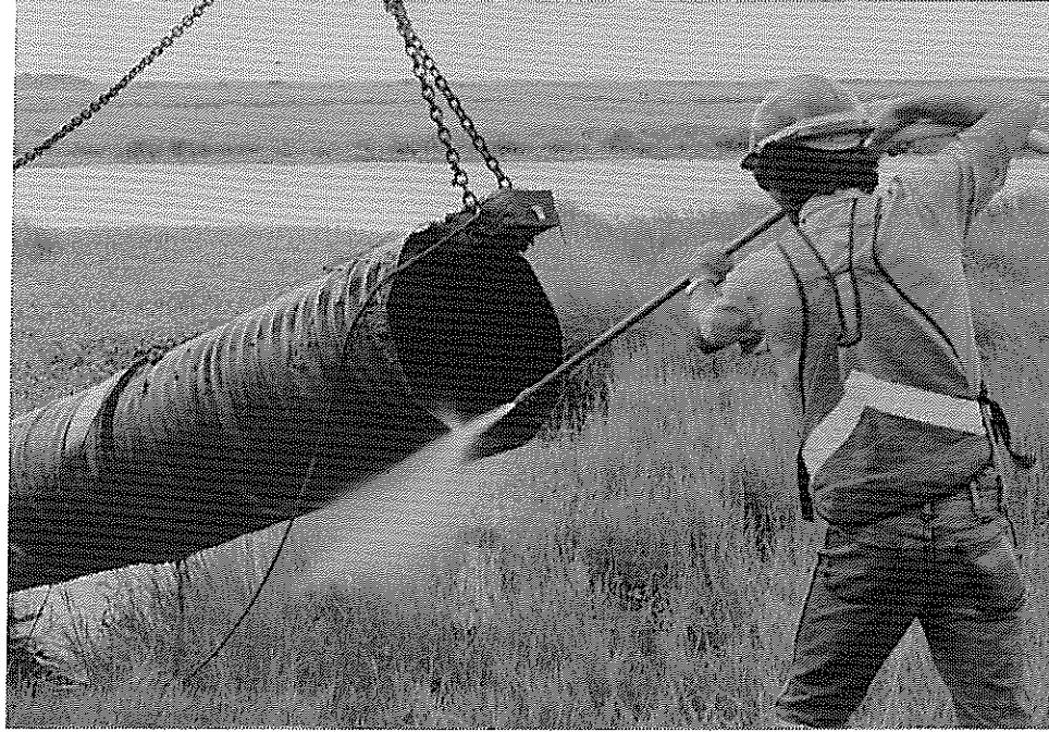
Figure 4. Each culvert is sprayed inside and outside with water.
