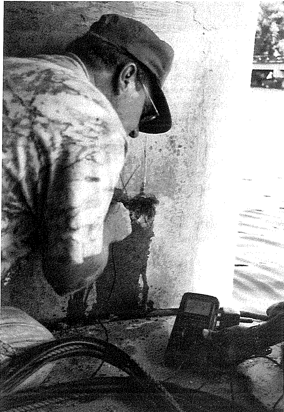
Figure 28 Half-cell potential test being conducted below the water
