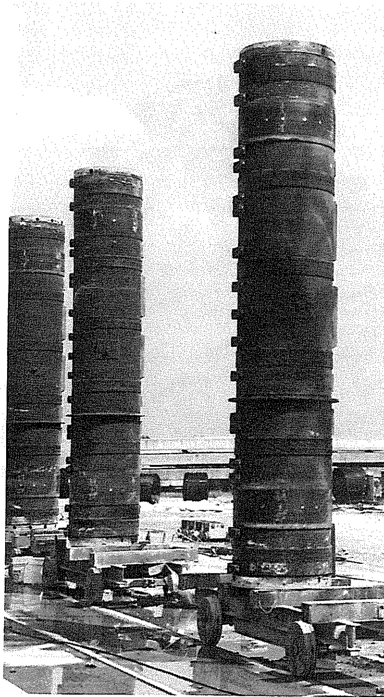
Figure 8 Pile segments being cured vertically
