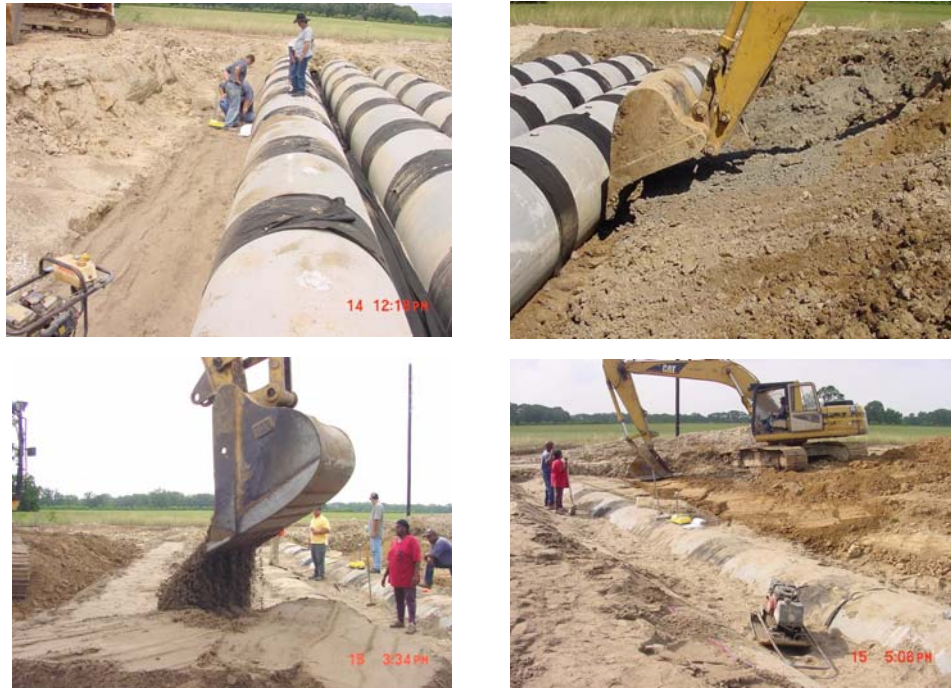
Figure 45 Example of backfill with transitional area
