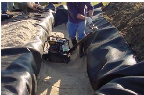
a. Compaction of sand at first lift
