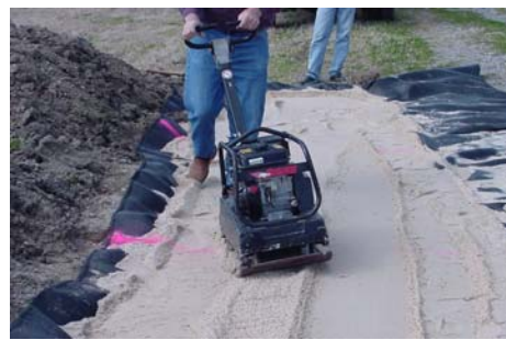
b. Compaction of sand at third lift
