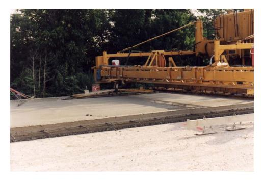
Figure 7 Finished surface of Portland cement concrete pavement
