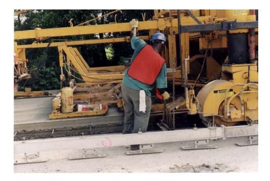
Figure 6 Placement of tie bars in the finished concrete pavement
