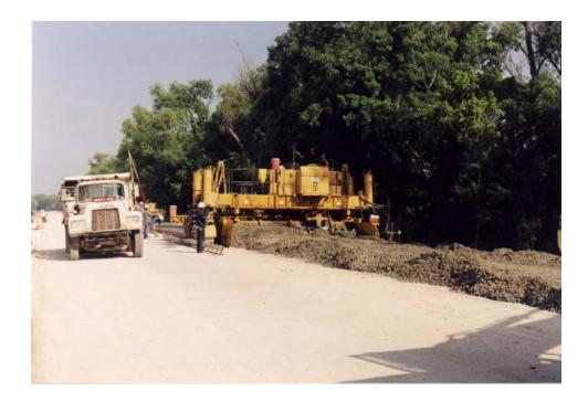
Figure 4 Slip form paver utilized during construction
