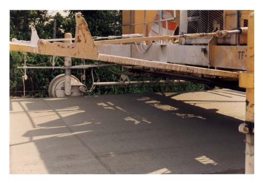
Figure 9 Creating macrotexture of concrete pavement surface by tining
