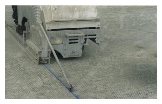
Figure 14 The early entry dry cutting of the narrow joints at test section S2
