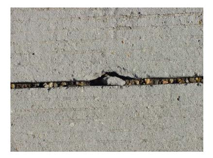
Figure 23 Low severity spalling of unsealed narrow contraction joints at test section S3
