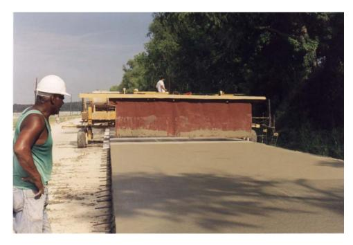
Figure 8 Creating microtexture of concrete pavement surface by use of burlap drag
