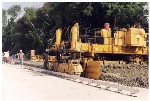
Figure 5 Detail of slip form operations
