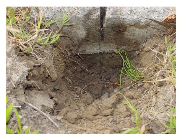
Figure 20 Verification of the development of the controlled crack across the narrow transverse contraction joints
