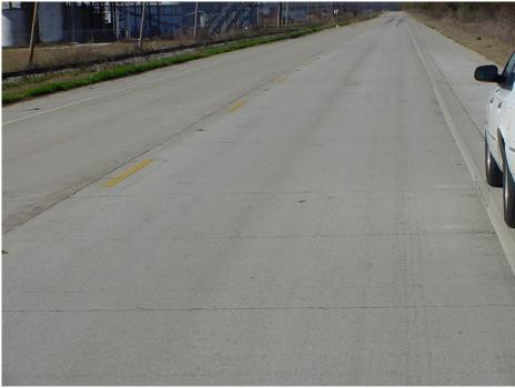
Figure 10 The new jointed plain concrete pavement at Northline Road
