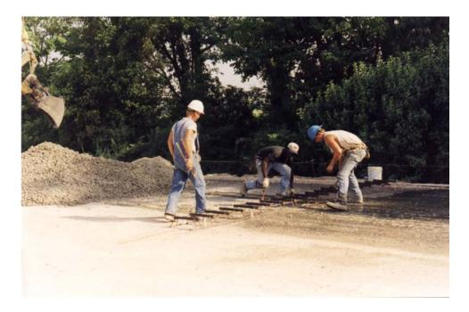
Figure 3 Placement of load transfer (dowel bars) at the transverse contraction joint location
