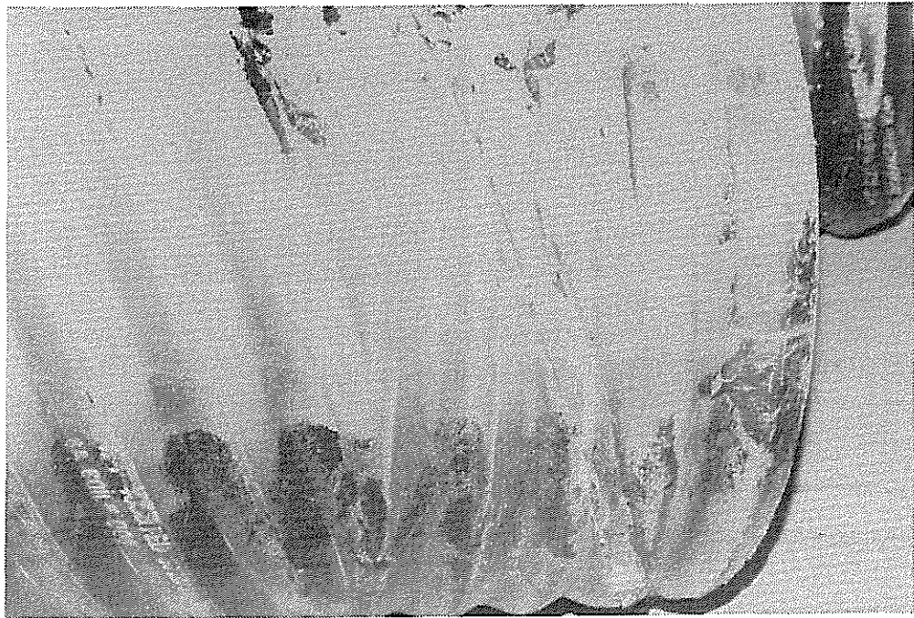
Figure G-15. This view shows very little white powder on the outside of the culvert.
