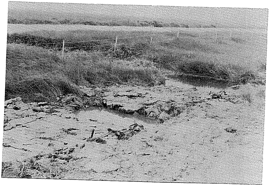
Figure 16. This is what the unprotected site looked like after the installation was completed.
