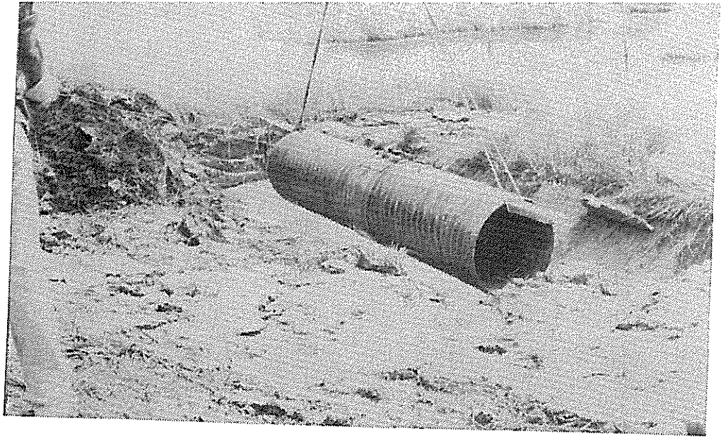
Figure 15. The unprotected culvert is lowered into the ditch.
