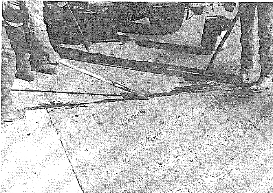
Removing excess joint seal material.
