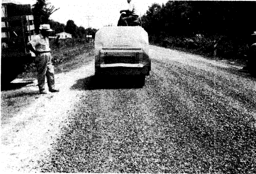
Figure xx 4 First Application Aggregate During Rolling with EA-2, Emulsified Asphalt.
