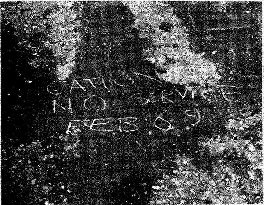
Photograph No. 2: RS-3K Treated Crack on New Orleans Service Road During February 1969
