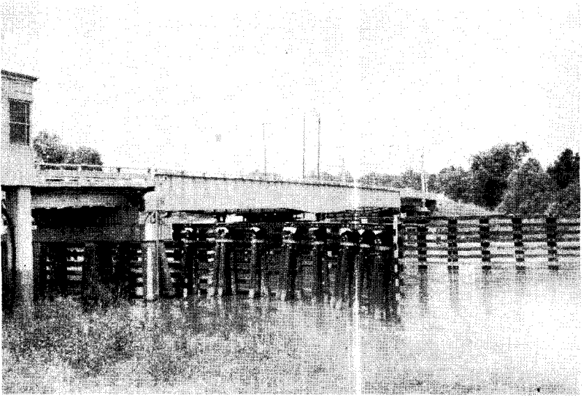
Figure No. 1: Overall View of Bridge No. 1
