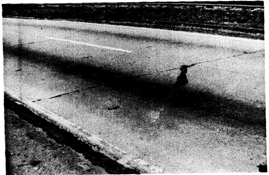
FIGURE 34 Slab Breakage
