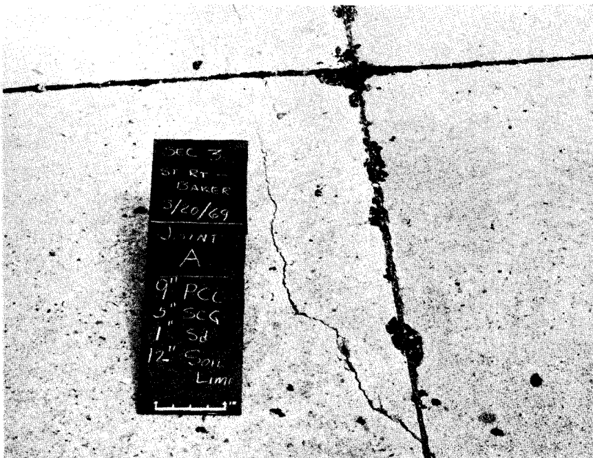
FIGURE 25 Pavement Spall
