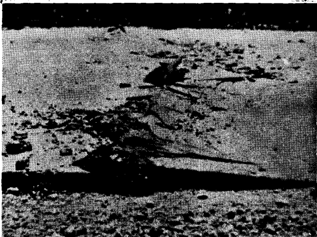
FIGURE 27 Pavement Blow-up
