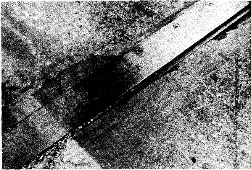
FIGURE 12 Typical Sliding Plate Joint
