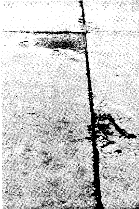
FIGURE 26 Pavement Spall
