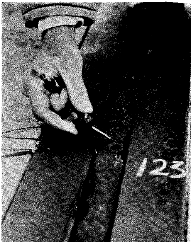
FIGURE 35 Failure Due to Truck Flare
