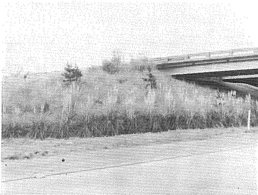
Figure 10. Slope stabilization with exotic vegetation. At this locality S1 in Calcasieu Parish in the I-10 study area, pampas grass has been successfully used to stabilize a repaired slope.
