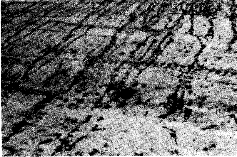
Figure 6 Closeup View Slope No. 5 at 1 Month
