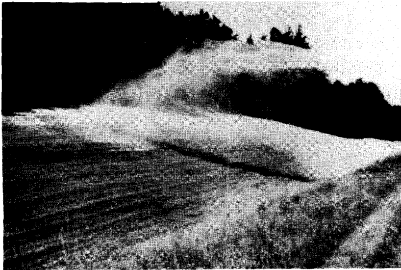
Figure 7 Installation of Product on Slope No. 1B
