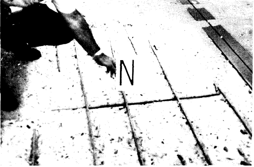
FIGURE 65 PRIOR TO PLACEMENT
