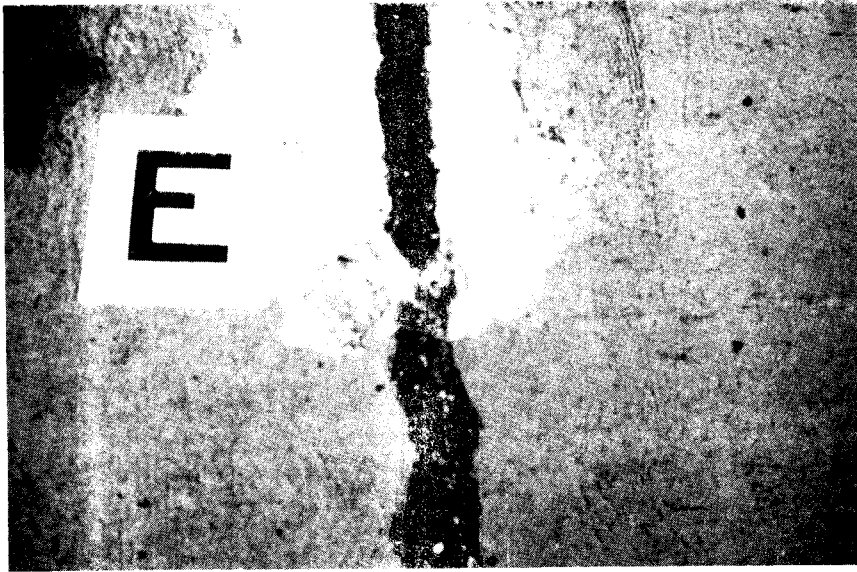
FIGURE 1 CONCRETE SURFACE AT STATION E-1
