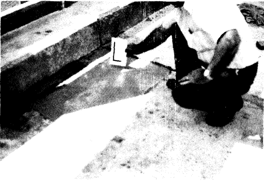
FIGURE 45 IMMEDIATELY AFTER PLACEMENT
