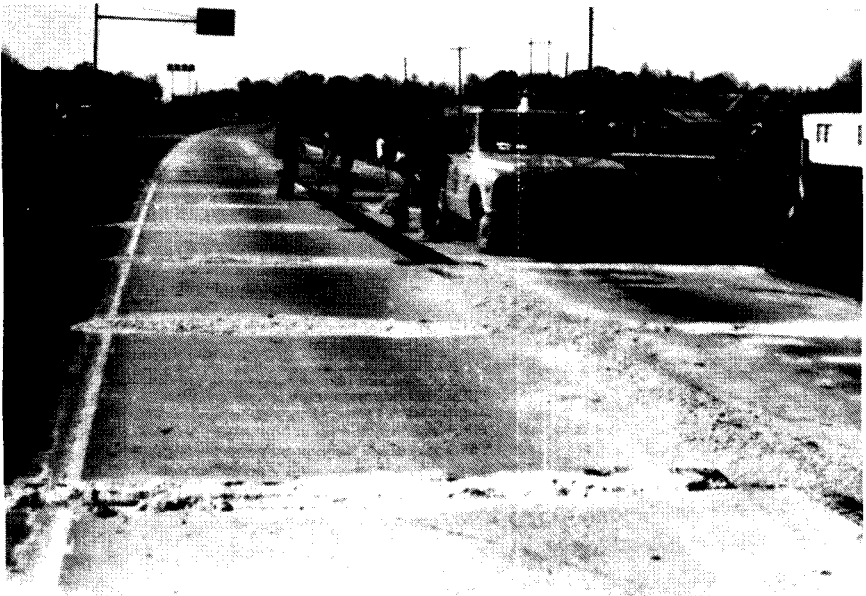
FIGURE 4 BLOTTING OF TACKED POLYPROPYLENE FABRIC
