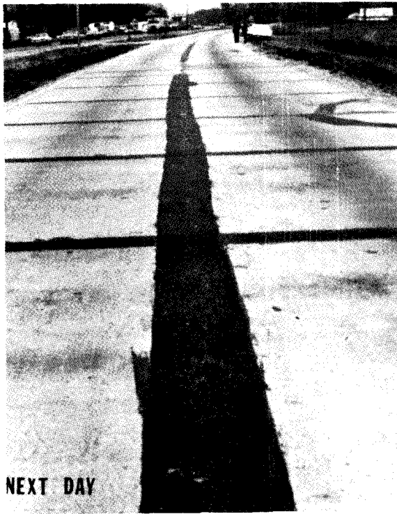
FIGURE 5 POLYPROPYLENE TEST SECTION PRIOR TO OVERLAY
