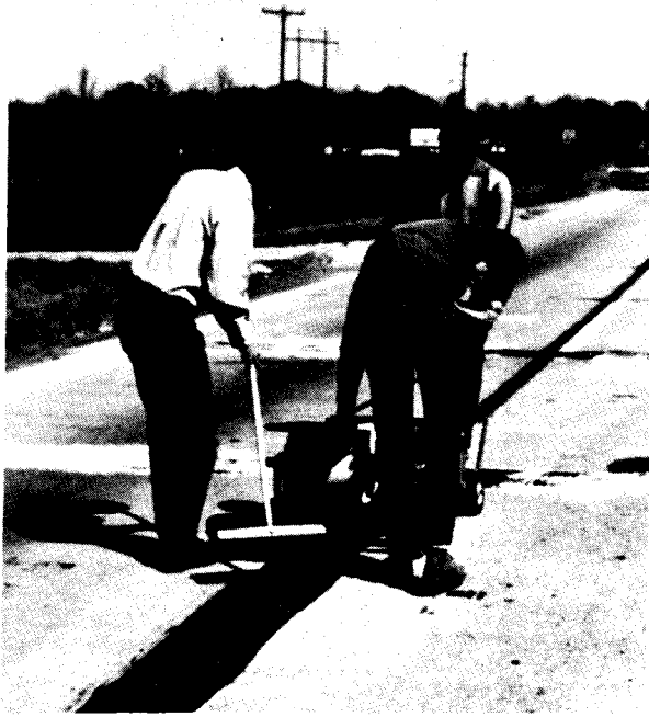
FIGURE 3 UNROLLING OF PRE-SOAKED POLYPROPYLENE FABRIC
