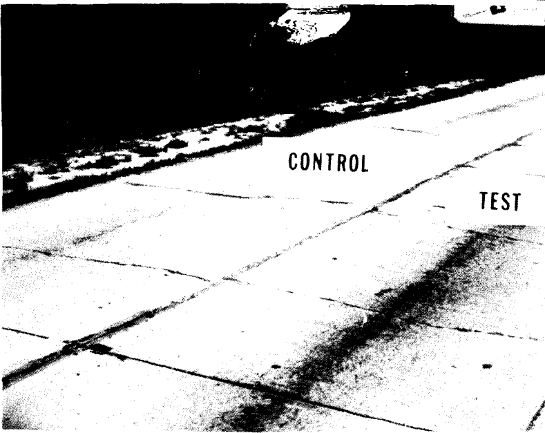
FIGURE I4 ORIGINAL CRACK PATTERN OF CONTROL AND TEST SECTION - LA. I9
