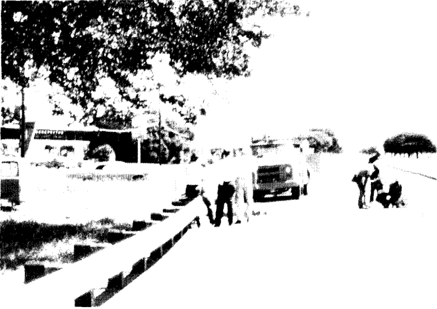
Figure 4 Site Chosen for WIM Installation
