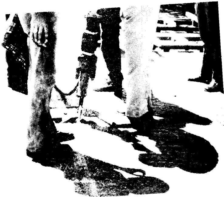
Figure 2 Removal of Material from Load Cell Calibration Area
