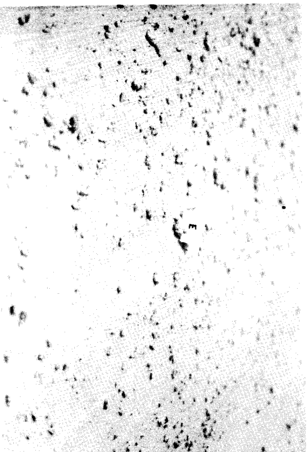
FIGURE 12 "Popcorning" on Longitudinal Texturing with Extra Heavy Nylon Broom
