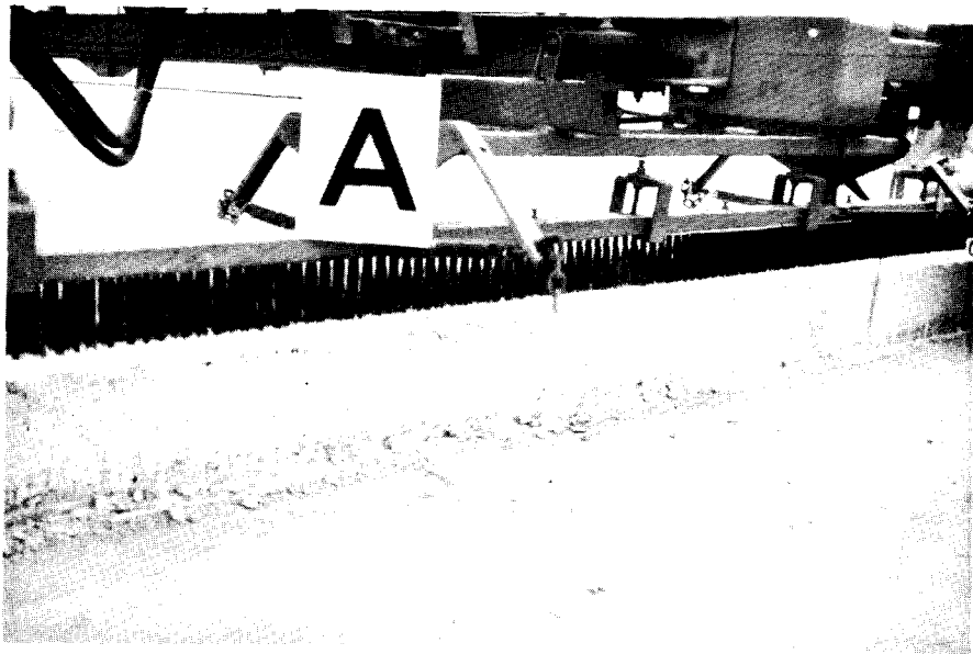
FIGURE 10 Heavy Polyplastic Broom on Transverse Texturing
