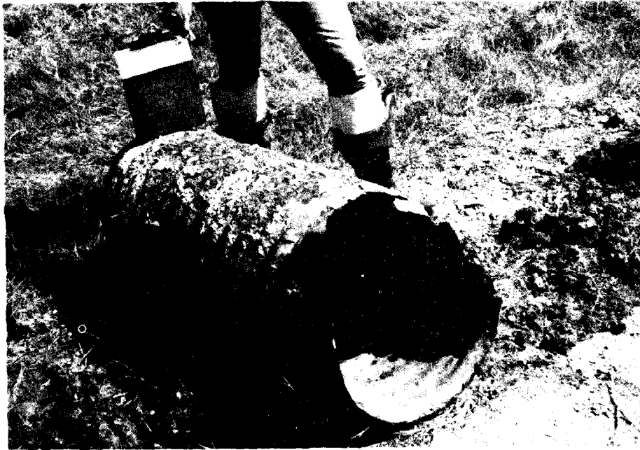
Galvanized Steel Culvert at Site No. 7 after Four Years FIGURE 3
